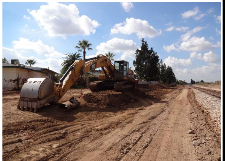
Grading work in Segment 4
