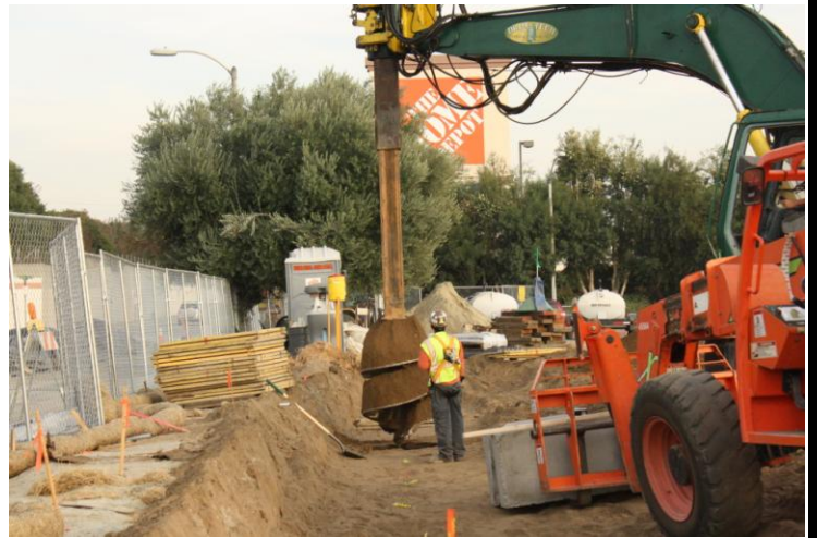
Soldier pile installation at Gold Line Operations Campus
