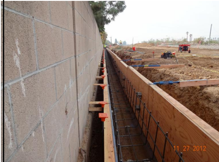
Drainage work at Citrus
