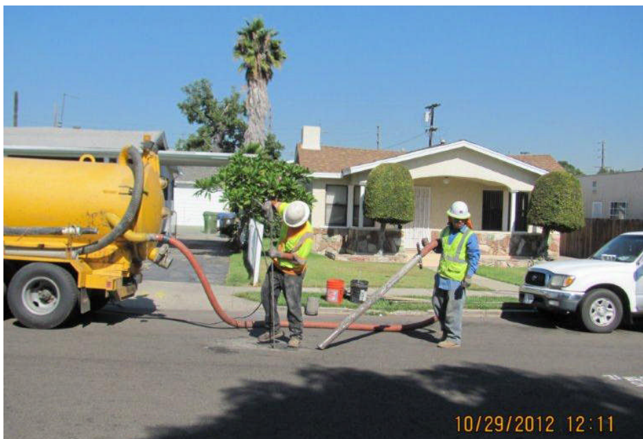
Crews locating utilities near 59 th Street.
