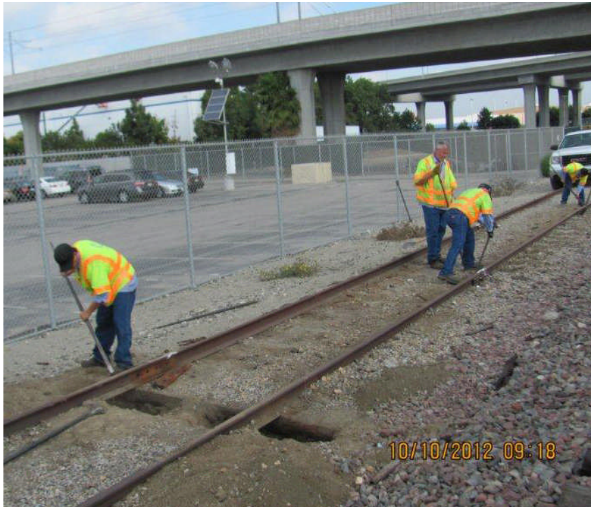
Track removal on Harbor Subdivision south of Imperial Highway.
