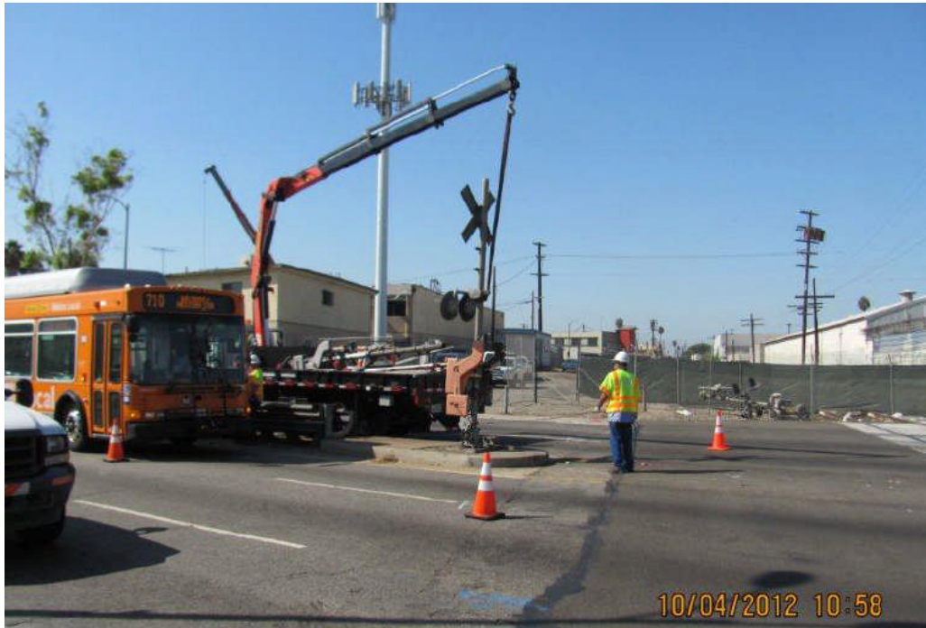
After BNSF abandonment process completed, crews remove Crenshaw St. railroad gate.
