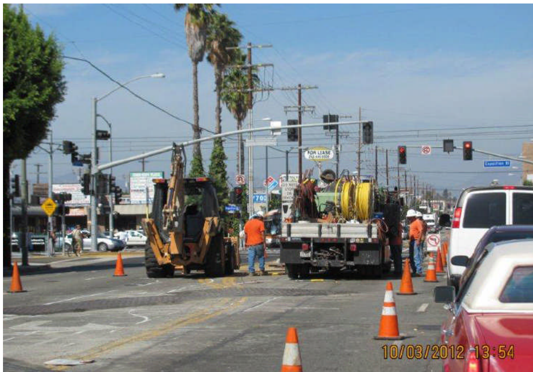
Gas Company utility relocation work at Crenshaw/Exposition Blvd.
