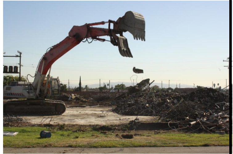
M&O Facility demolition
