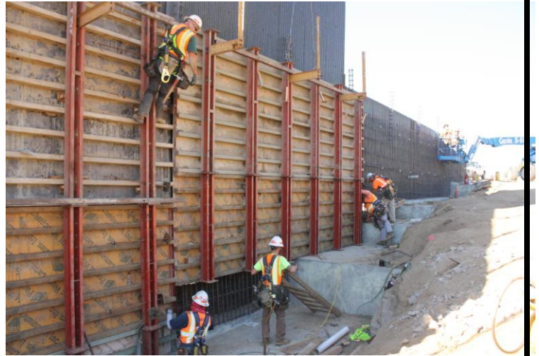
Construction of retaining walls
