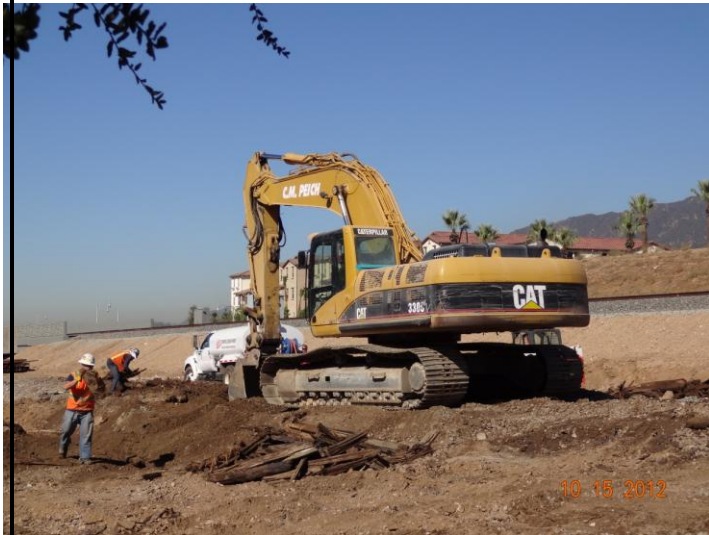
Alignment grading work
