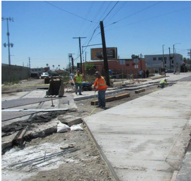
Dowel Placement on 67th .
