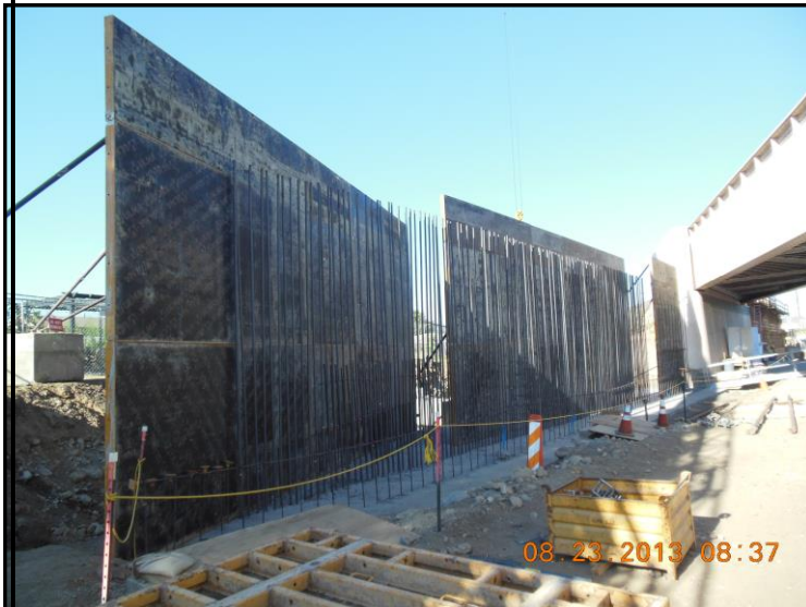
Segment 4: Foothill Bridge FRT Abutment 1
