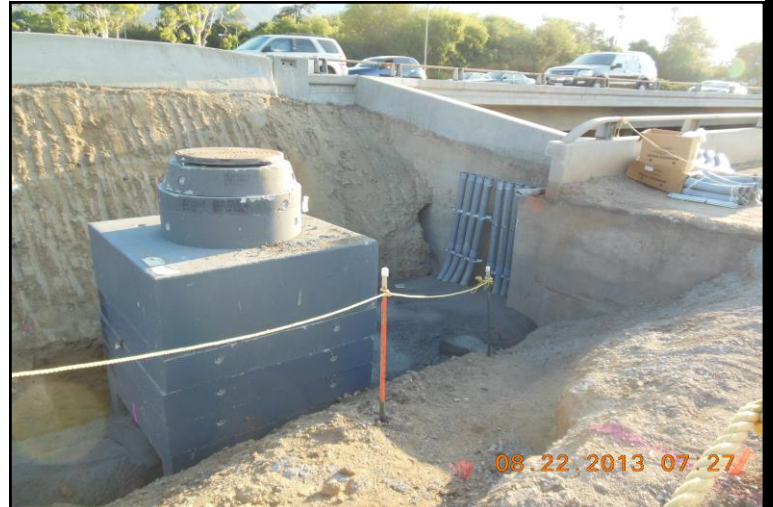
Segment 1: Conduit and vault work for traction power substation
