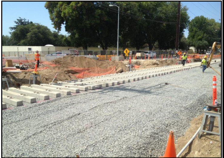
Segment 3: California Grade Crossing
