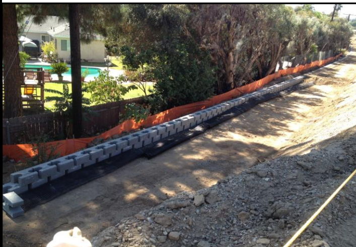
Segment 2: MSE Wall East of IFS
