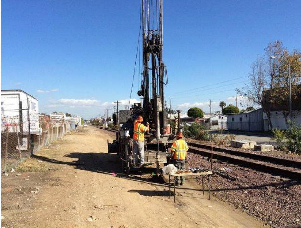
Geotechnical boring at a depth of 25 ft.
