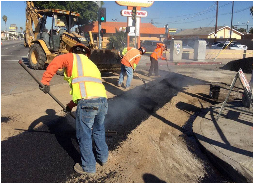
Asphalt paving on 67 th Street.
