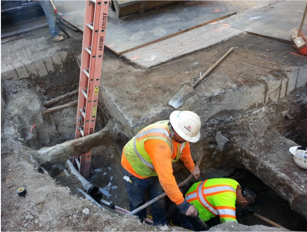
Sixth Street and Flower – Level 3 conduit installations by Irish Construction, Inc.
