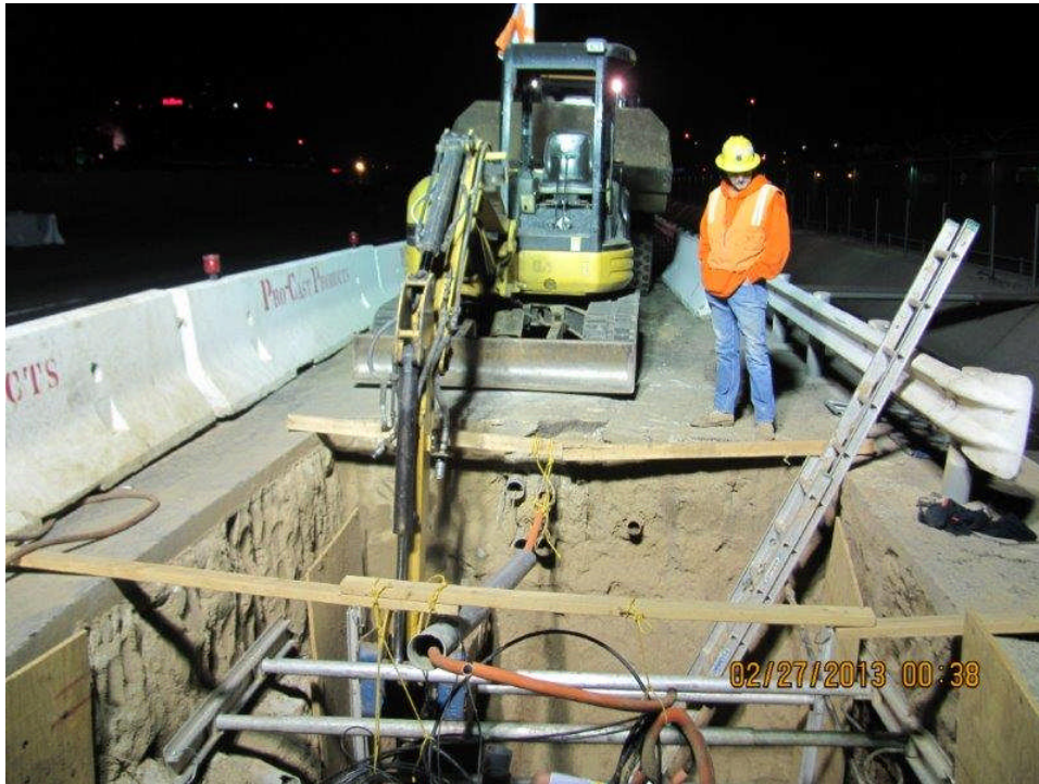
Removing manhole at LAX near Runway 25R.
