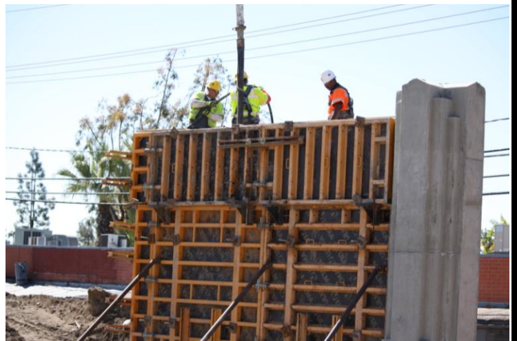
Work at Colorado Bridge
