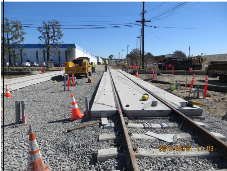
Track work at Highland grade crossing
