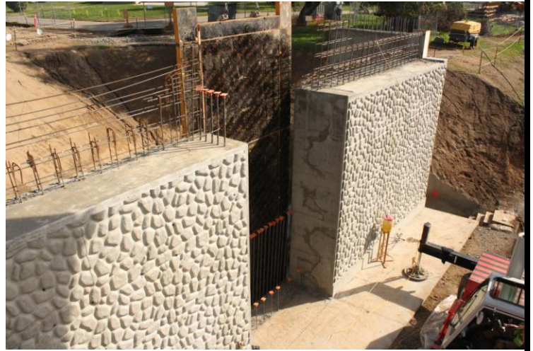
Work at Citrus Bridge
