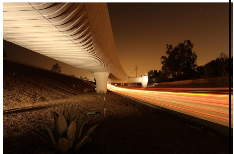
Nighttime view – soffit
