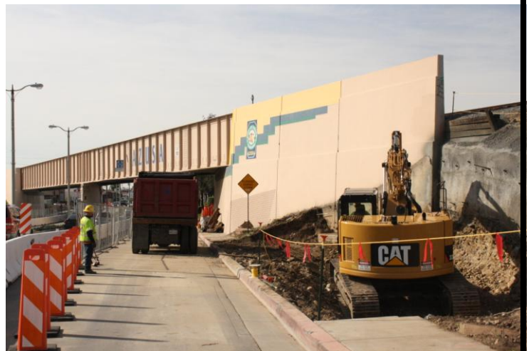
Work at Foothill Bridge
