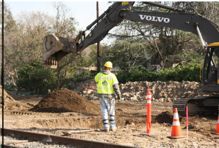
Grading in Segment 4
