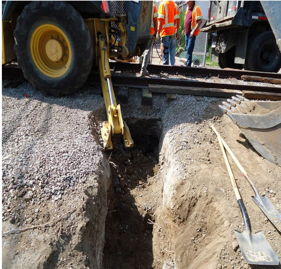
Advanced Utility Work on 96 th Street.
