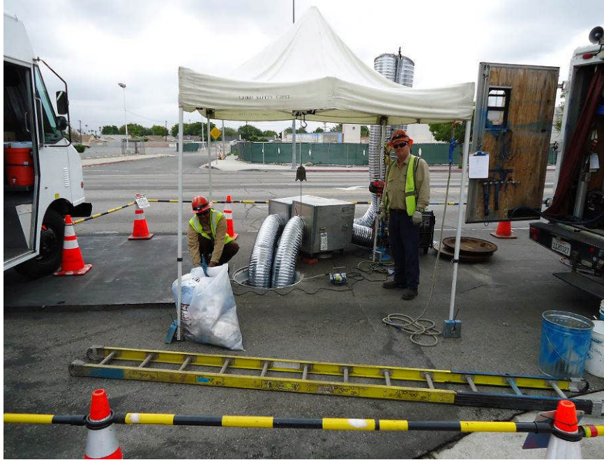
Advanced Utility Work by LADWP on Crenshaw Boulevard.
