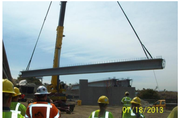
Precast Girder Erection at San Gabriel River Bridge
