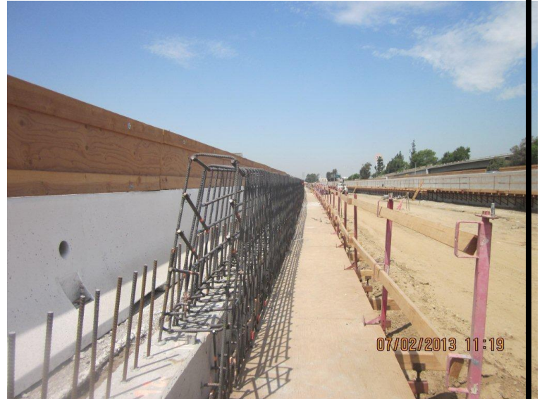
Barrier Wall Construction in Segment 1
