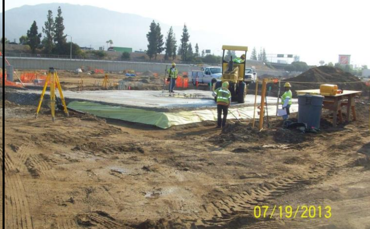
MOW building pad foundation base preparation
