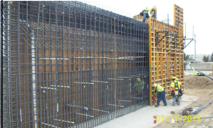
Santa Anita Bridge Abutment #3 Wall
