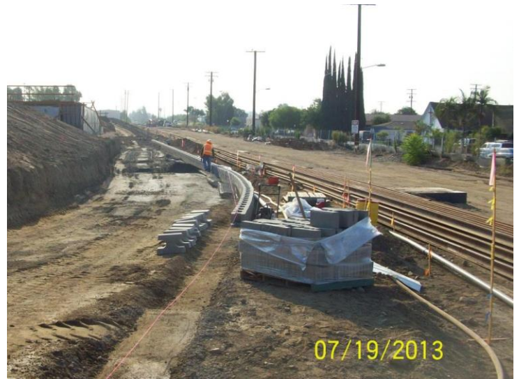
South Campus MSE Wall C
