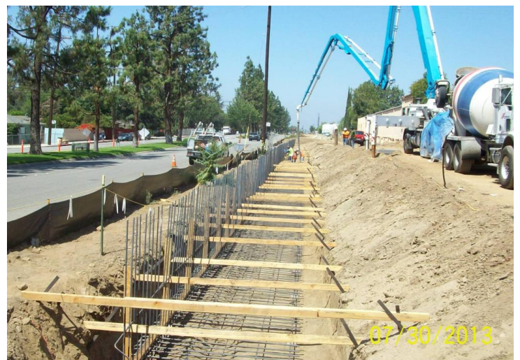
Duarte Road CMU retaining wall footing
