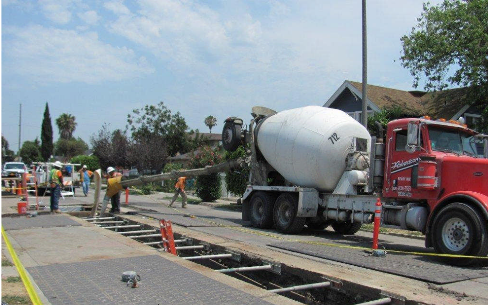
59 th Place concrete encasement.
