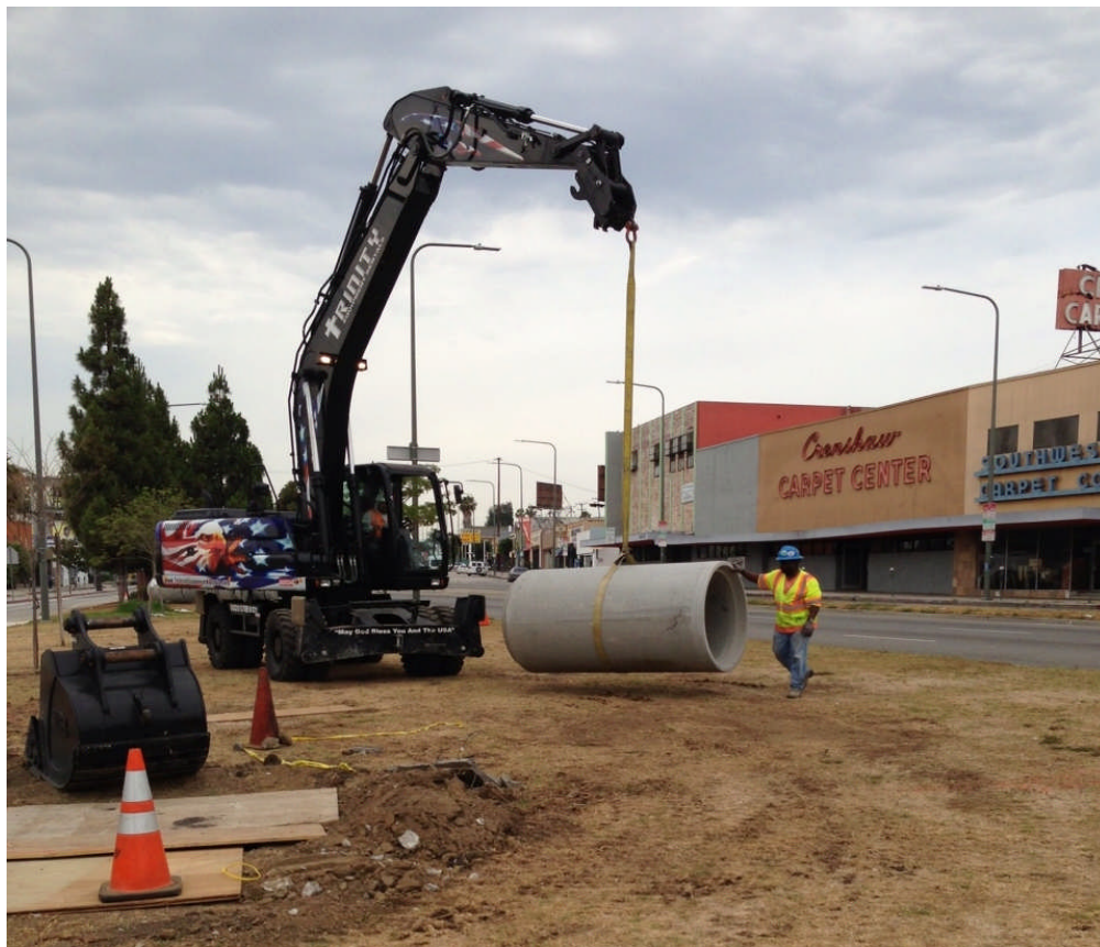
Leimert Park relocation of concrete pipe.
