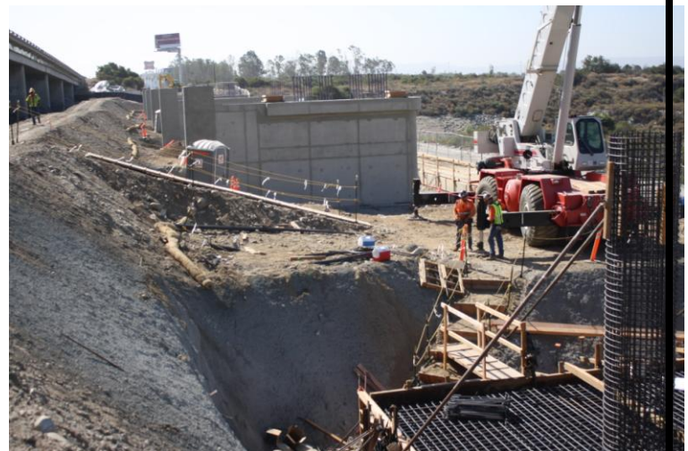
San Gabriel River Bridge
