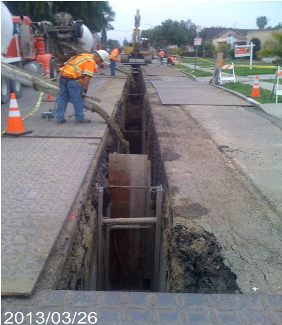
Advanced Utility Relocations contractor at 60 th St placing slurry.
