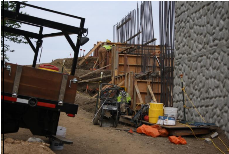
Work at Azusa-Citrus bridge
