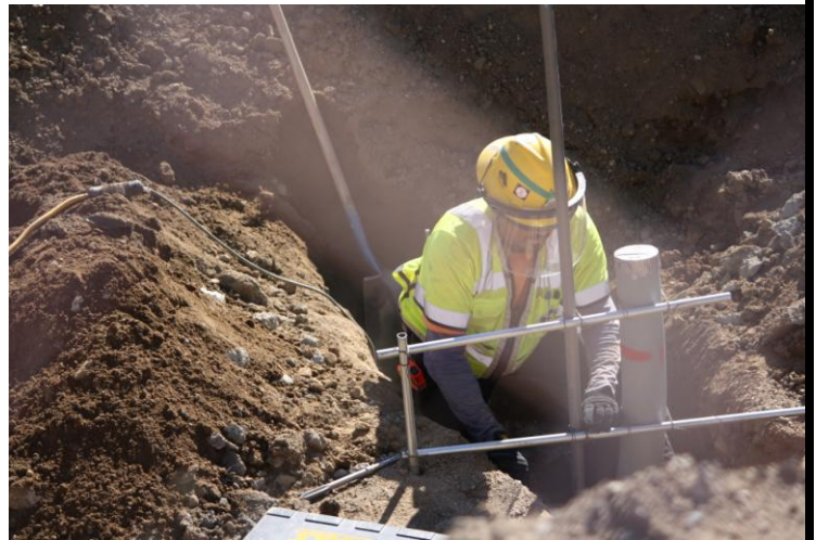
Duct bank work at Gold Line Operations Campus
