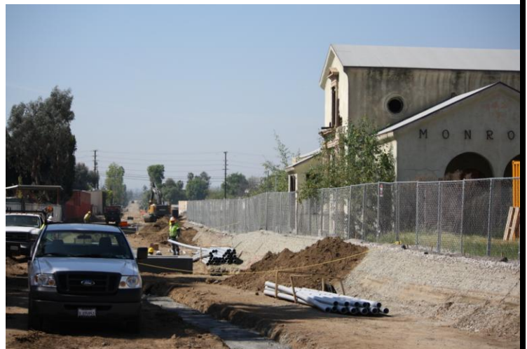
Excavation work at Monrovia Station
