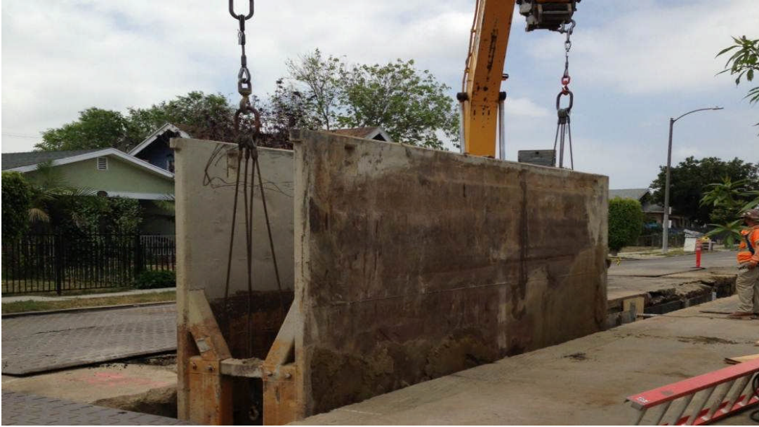
Advanced utility relocations contractor extracting shoring box.
