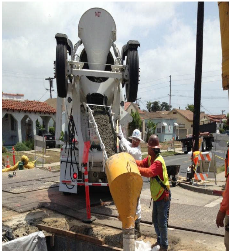
Advanced utility relocations contractor slurry pour on 60 th Street.
