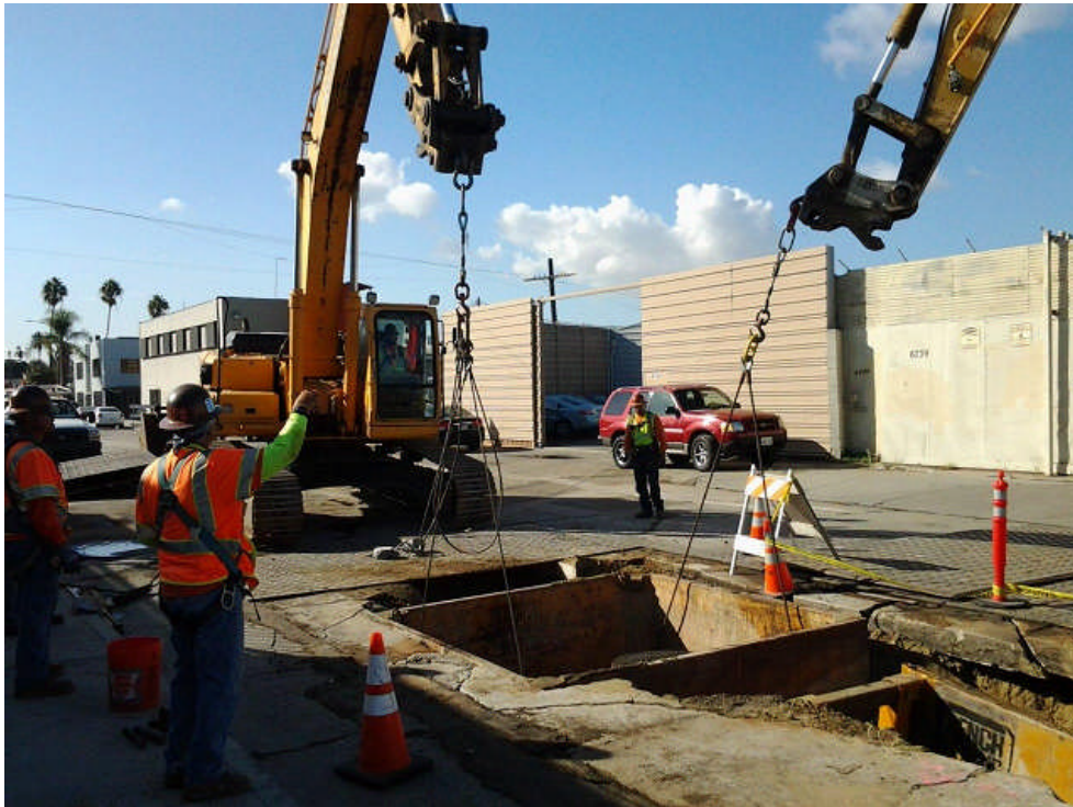
Advanced Utility Relocation sewer work on Victoria Avenue.
