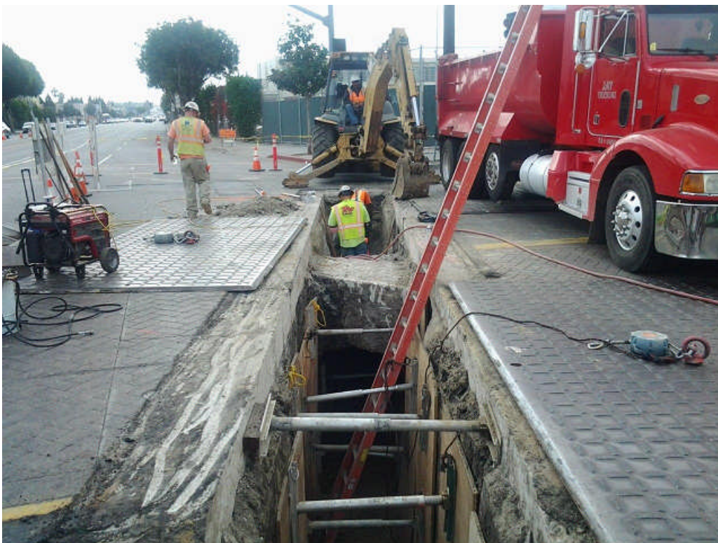
Excavation for 10" VCP Sewer on 60 th Street.
