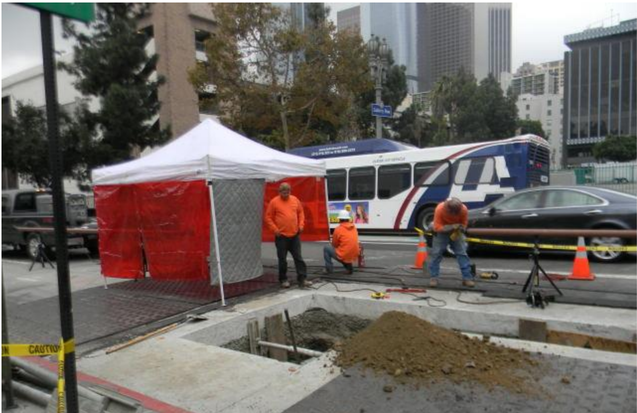
Gas Line Relocation at 2 nd Street and Spring
