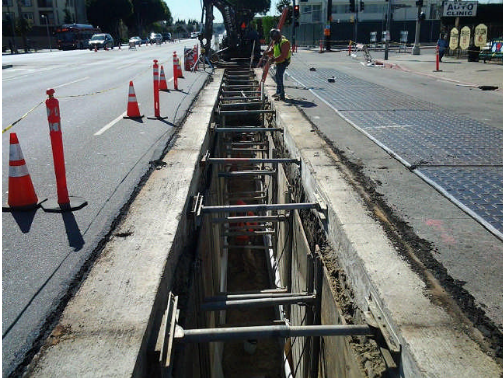
Excavation and shoring along Crenshaw Boulevard.
