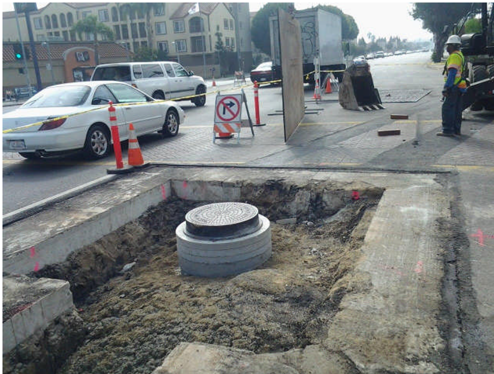
Slurry Backfill between 59 th and 60 th Street.
