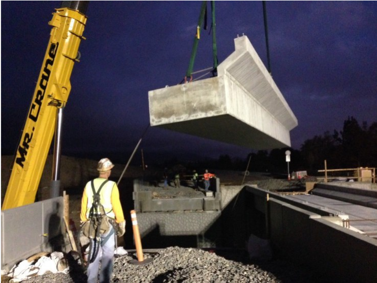
Segment 4 — Palm Ave Bridge Girder Installation
