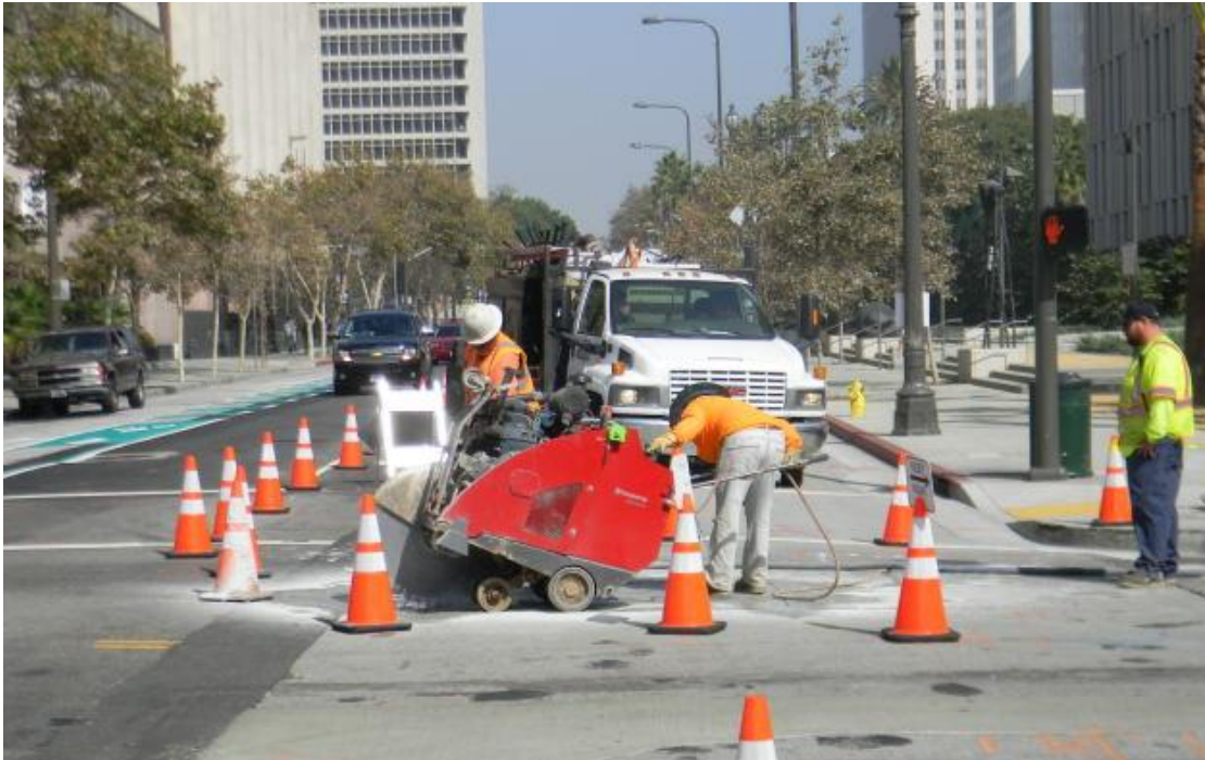
SE Pipeline Saw Cutting at 2 nd and Spring
