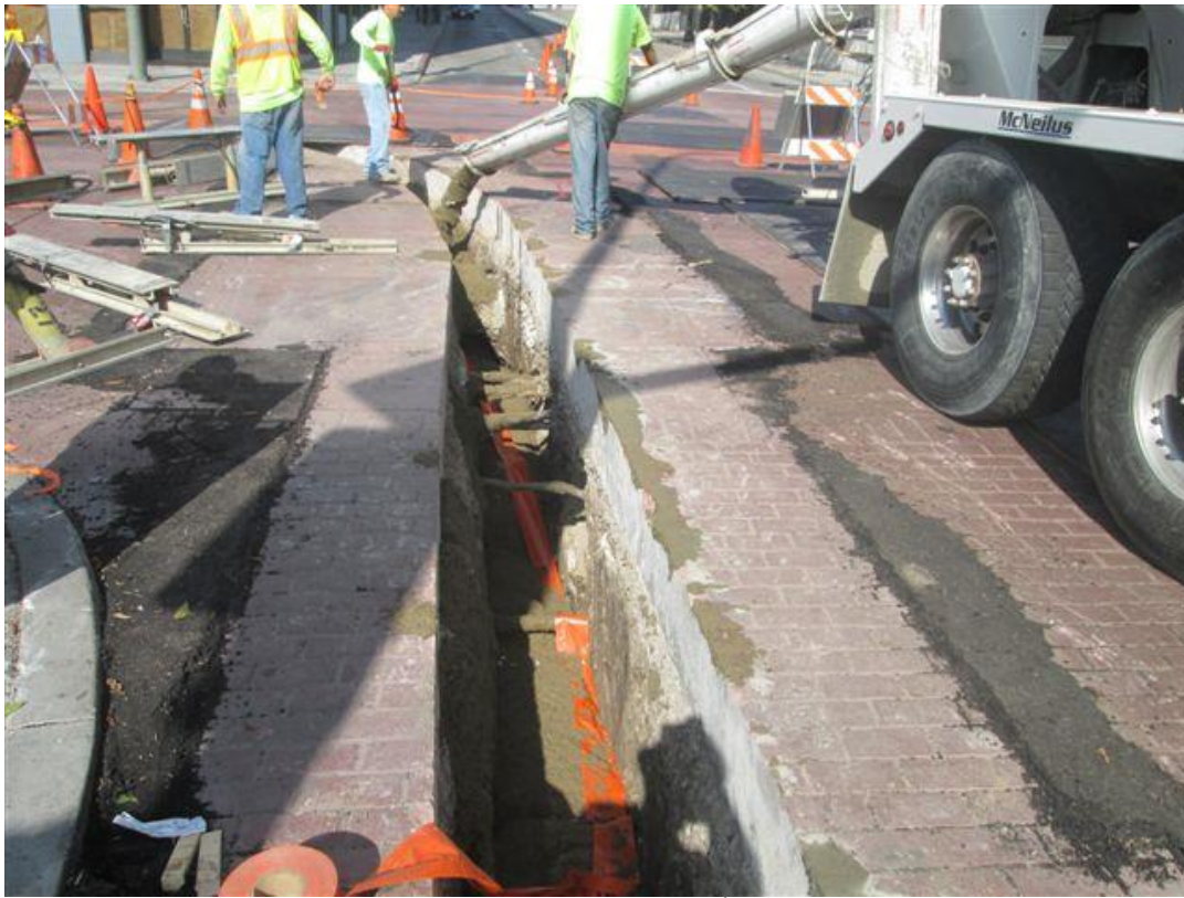
TWC Joint Trench Work at 2 nd and Broadway
