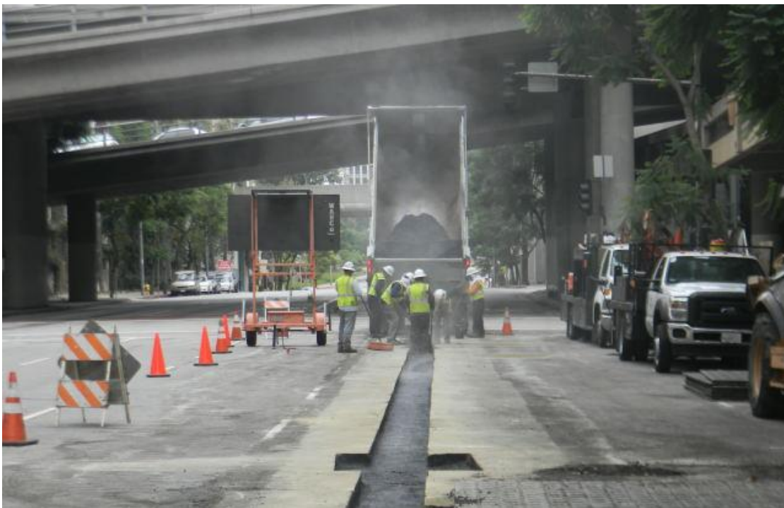
Paving 3" Gas Line Trench at Flower Street
