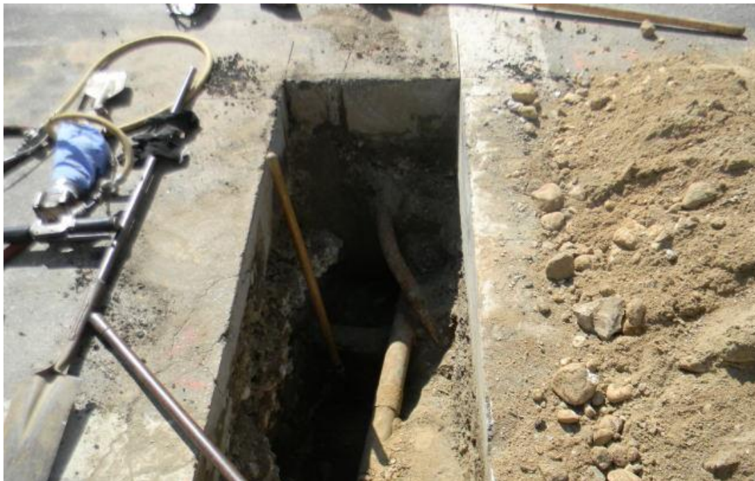
SE Pipeline 2 nd Street Potholing
