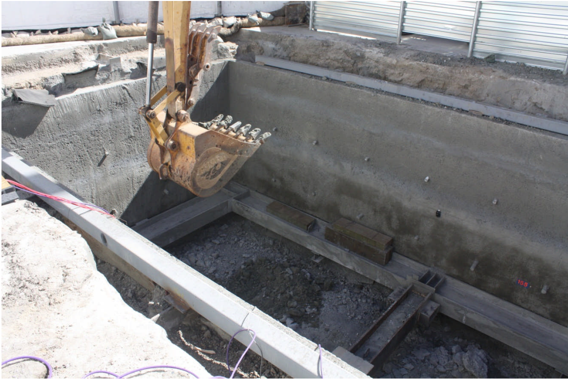
Excavation of the Exploratory Shaft
