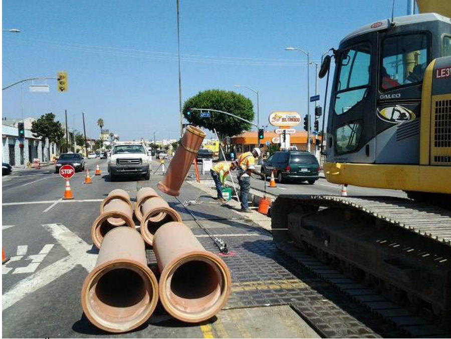
67 th /Crenshaw installation of 18" Vitrified Clay Pipe (VCP).
