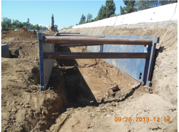
Excavation for Final CMU Wall in Segment 1
