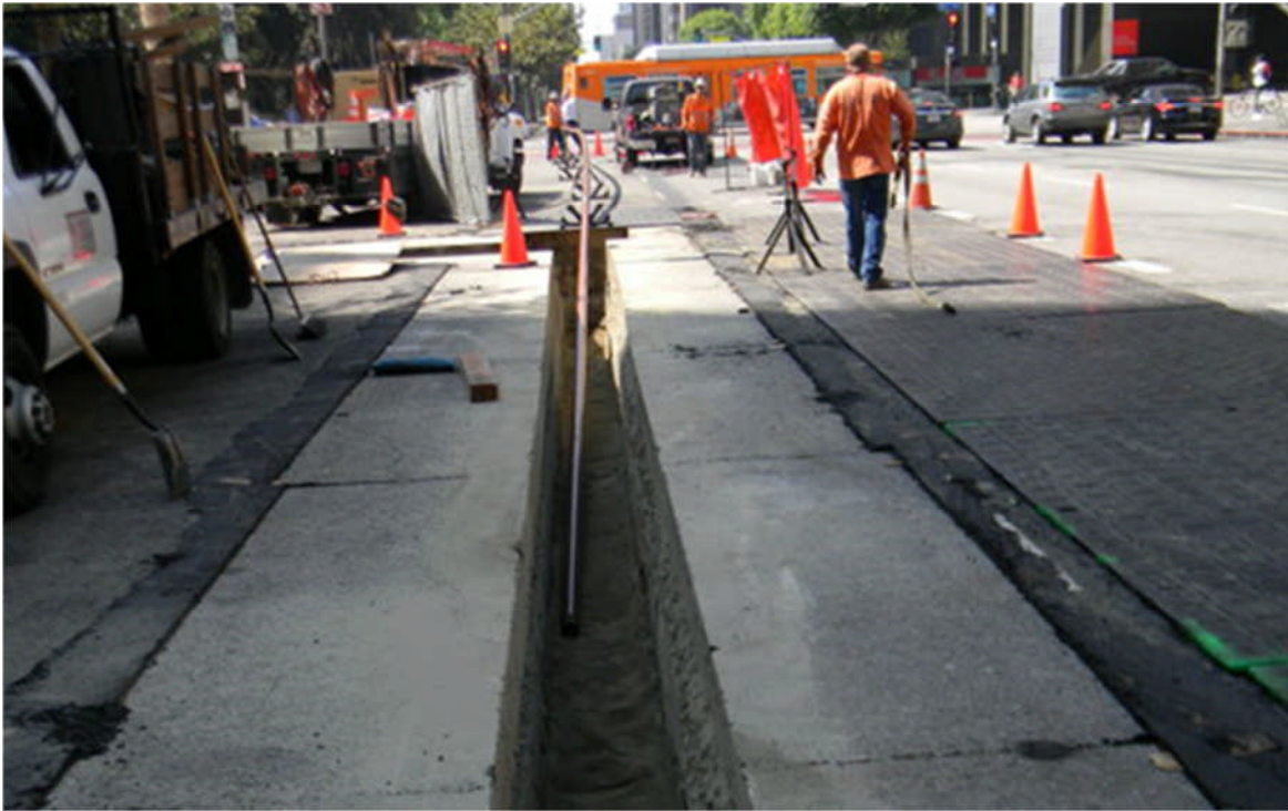
New 3" Gas Main Being Placed into Trench on Flower Street.
