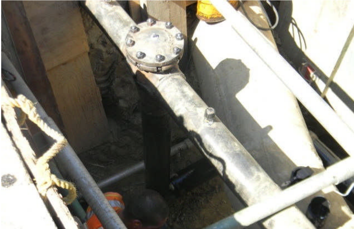
New 6" Gas Line at Hope Street.
