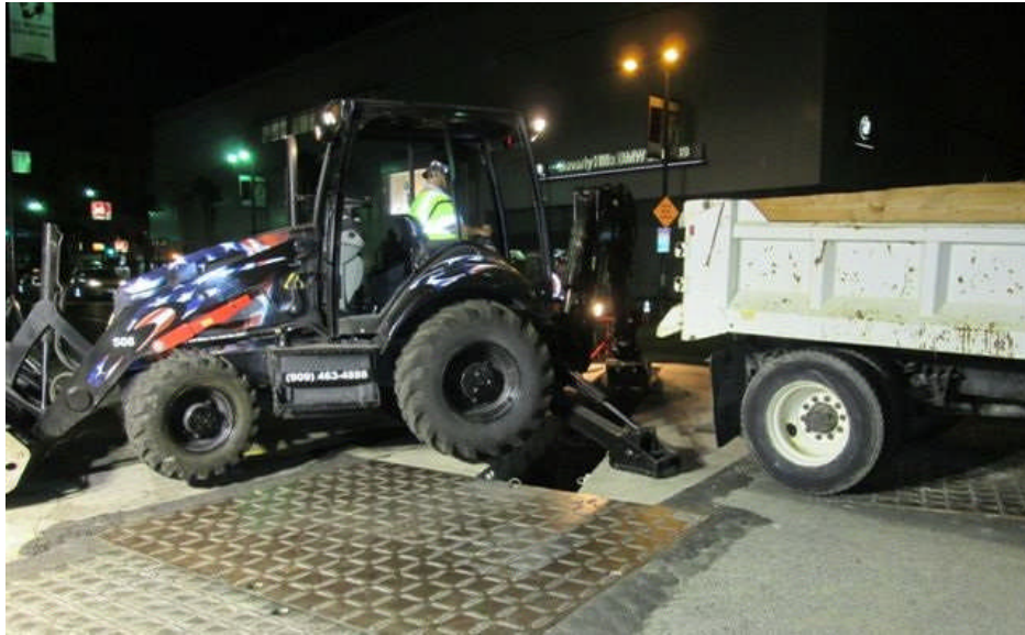
Utility potholing at Wilshire Blvd. and Orange
