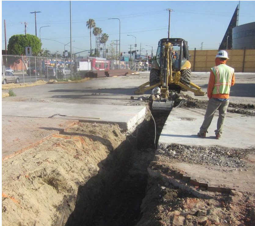
Pre trenching for SOE wall section.
