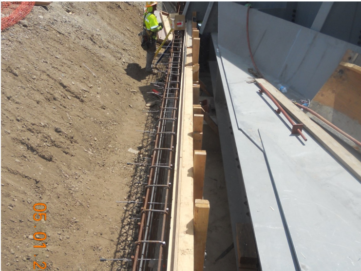
Segment 4: Foothill Bridge - Backwall Construction
