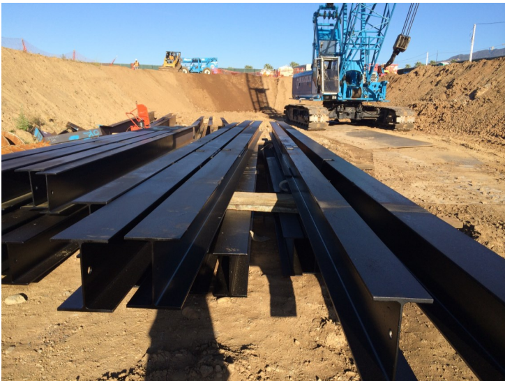
Soldier Beams at Azusa-Citrus Parking Structure
