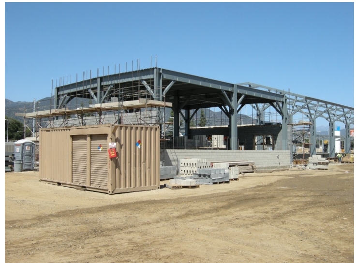
Operations Campus: MOW Storage Building Exterior CMU Work
