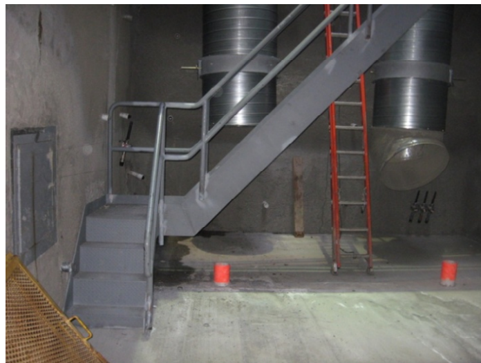
View of Bottom Level of the Exploratory Shaft
