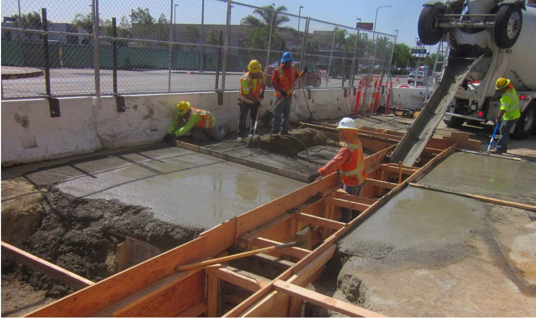
Placing slurry to stabilize CSM trench.
