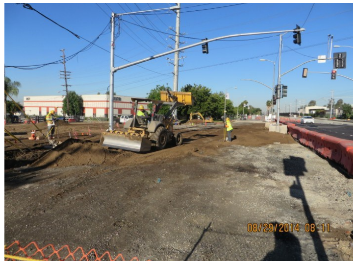
Segment 3: Mountain Ave - Rough Grading
