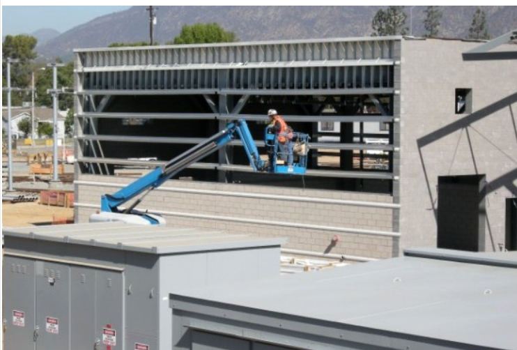
Operations Campus: MOW Storage Building - Metal Siding
