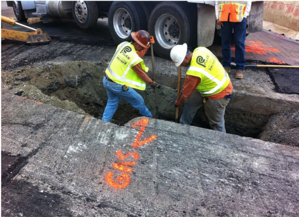
DWP Power Trench at the corner of Flower St. and 5 th .
