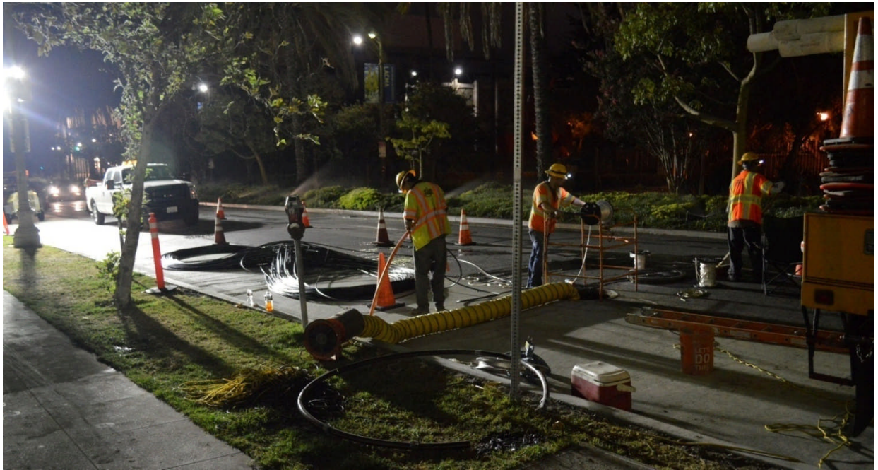
CES Performing Fiber Optic Work on Wilshire Boulevard in the City of Beverly Hills
