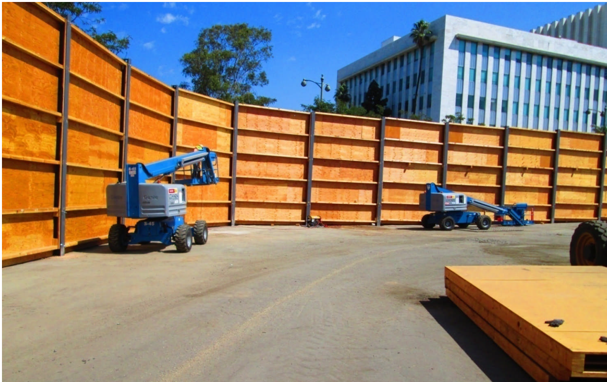
Installation of Sound Wall at the Wilshire/Crenshaw Laydown Yard
