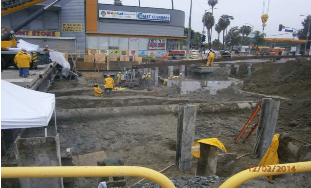
Continued excavation on deck beam 44 and 45 area at the Expo Station.
