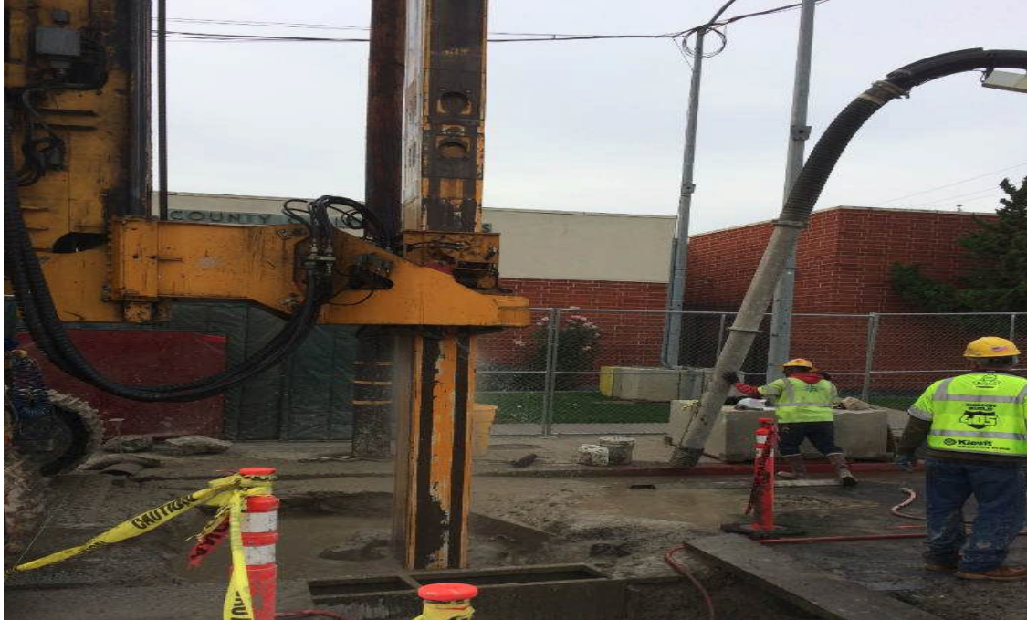
Expo North Headwall Drilling CSM Panel N1.
