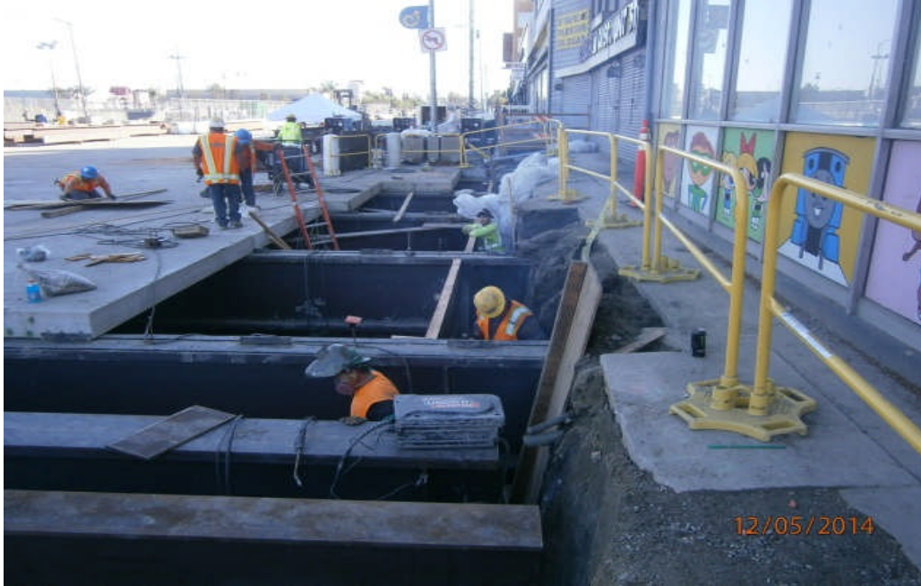
Formed and Placed Slurry on west side of excavation.
