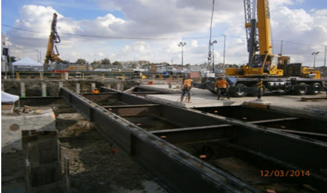
Continued to place concrete deck panels.
