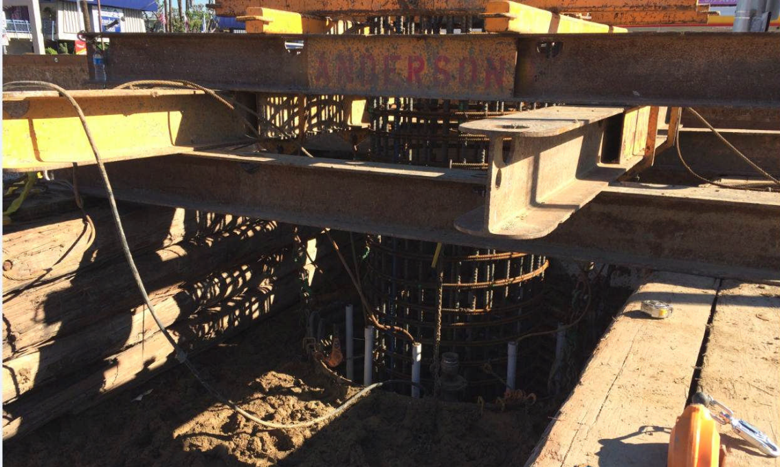
Aviation/Century Aerial Structure Bent 4R CIDH Pile and Column Cage.
