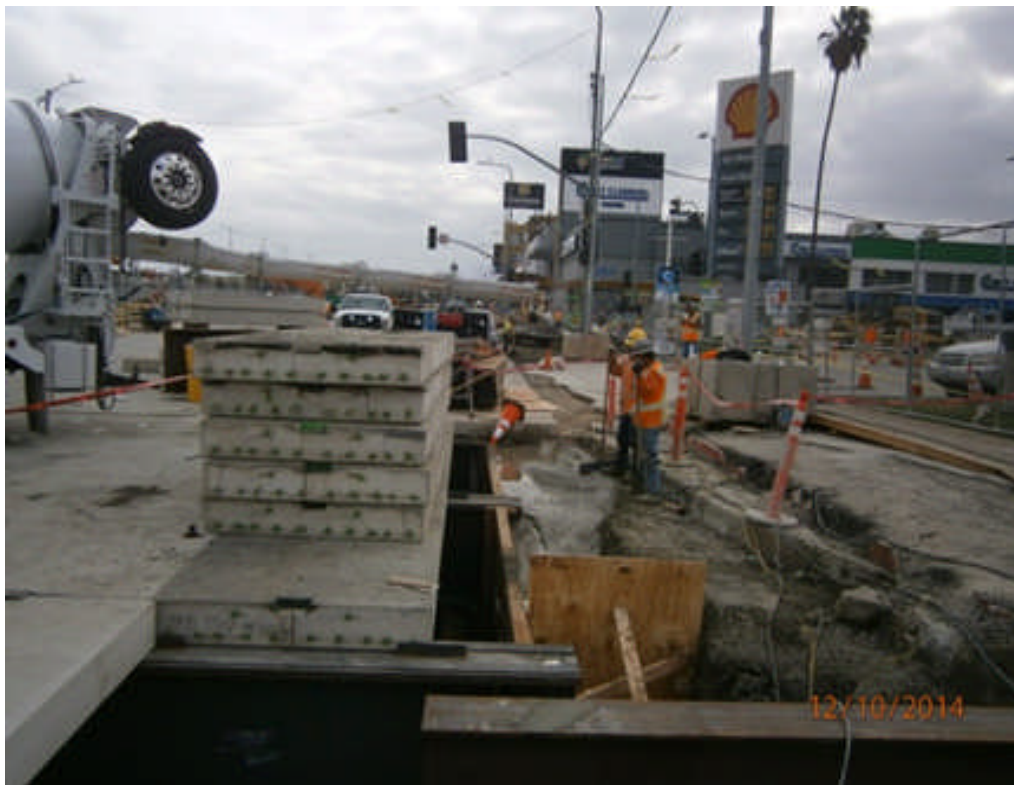
Slurry Backfill on outer edges of excavation north of Rodeo Road.
