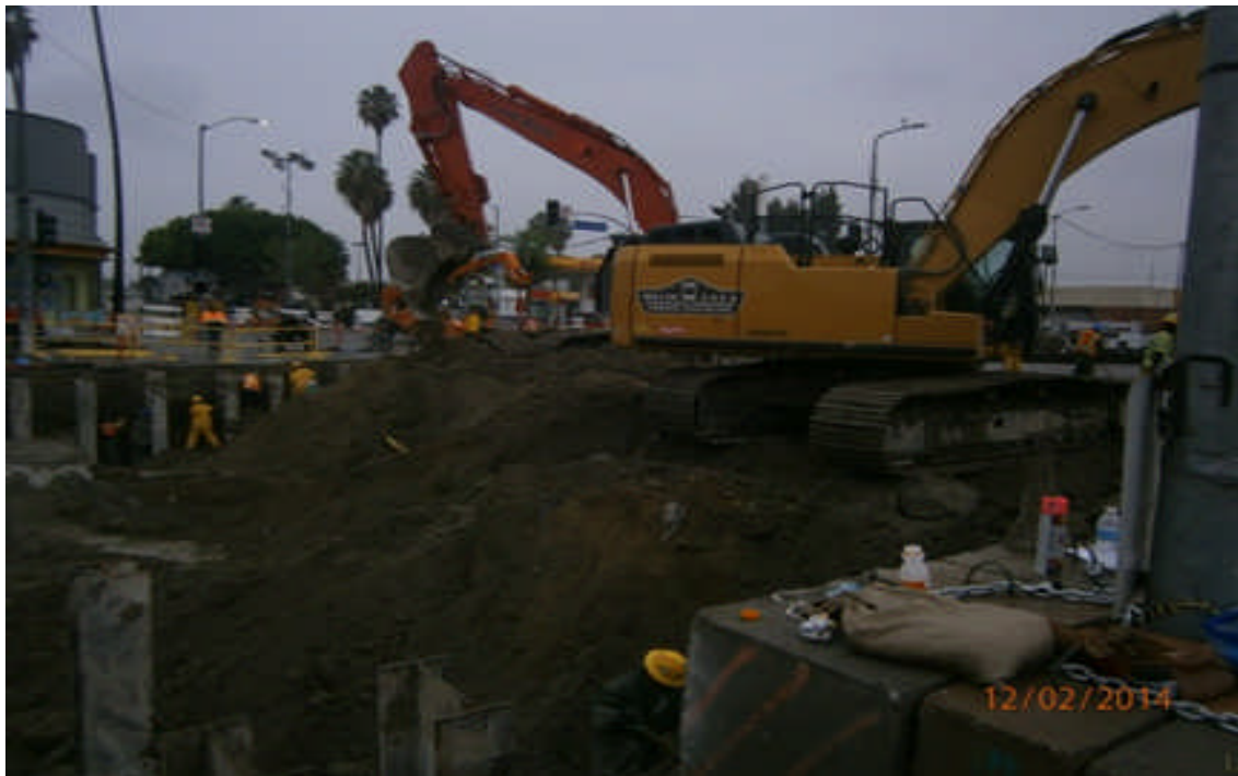
Excavation of Expo Station at beam 45, 46 and 47 area.
