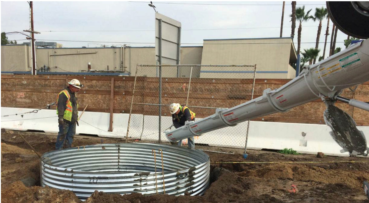
Aviation Century Aerial Structure Bent 8R CMP Isolation Casing.
