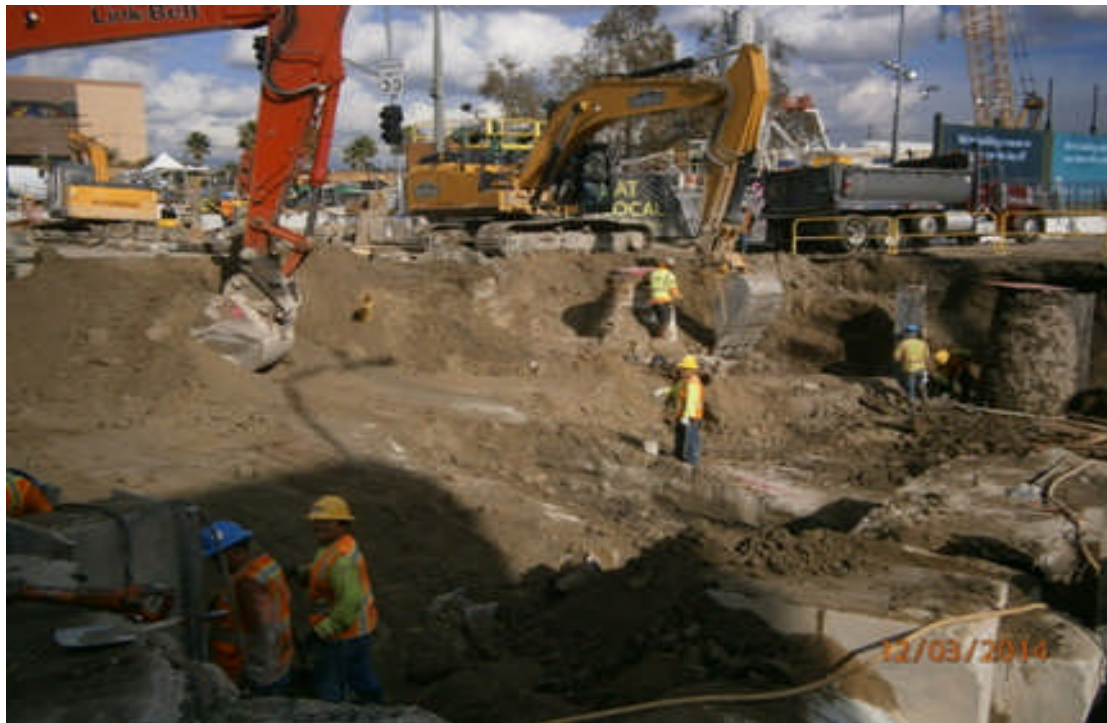
Continued excavation of beams 48 and 49 areas.
