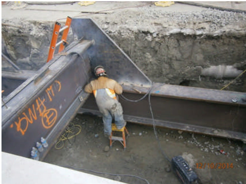
Welding on Deck and Cap Beams at Crenshaw and Rodeo.
