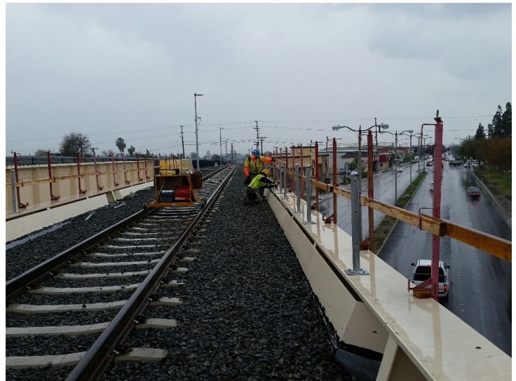
Segment 4: Foothill Bridge Cable Installation
