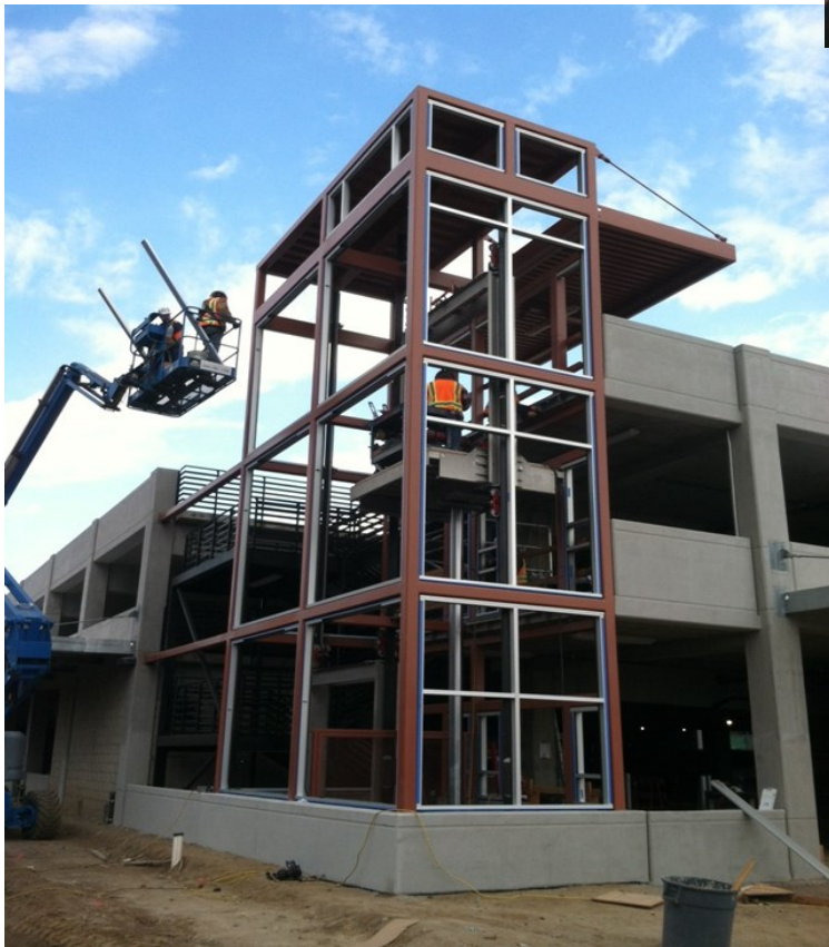
Monrovia Elevator - Steel Framing Installed
