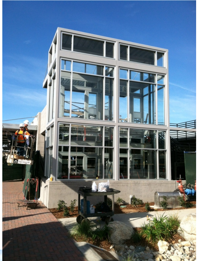
Arcadia Elevator - Glass Installation Complete
