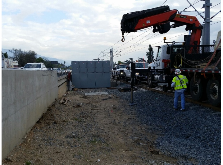
Segment 1: Michillinda TPSS Cabinet Installation
