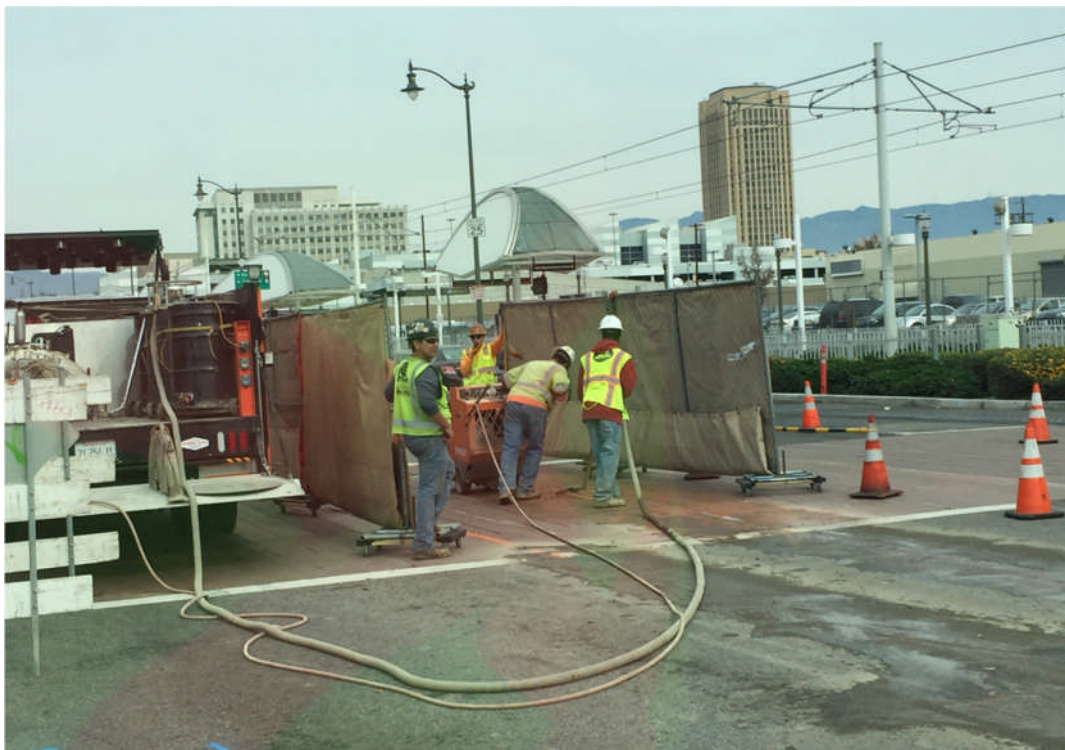
AUR C0981R – Saw cutting using sound blanket along Alameda Street
