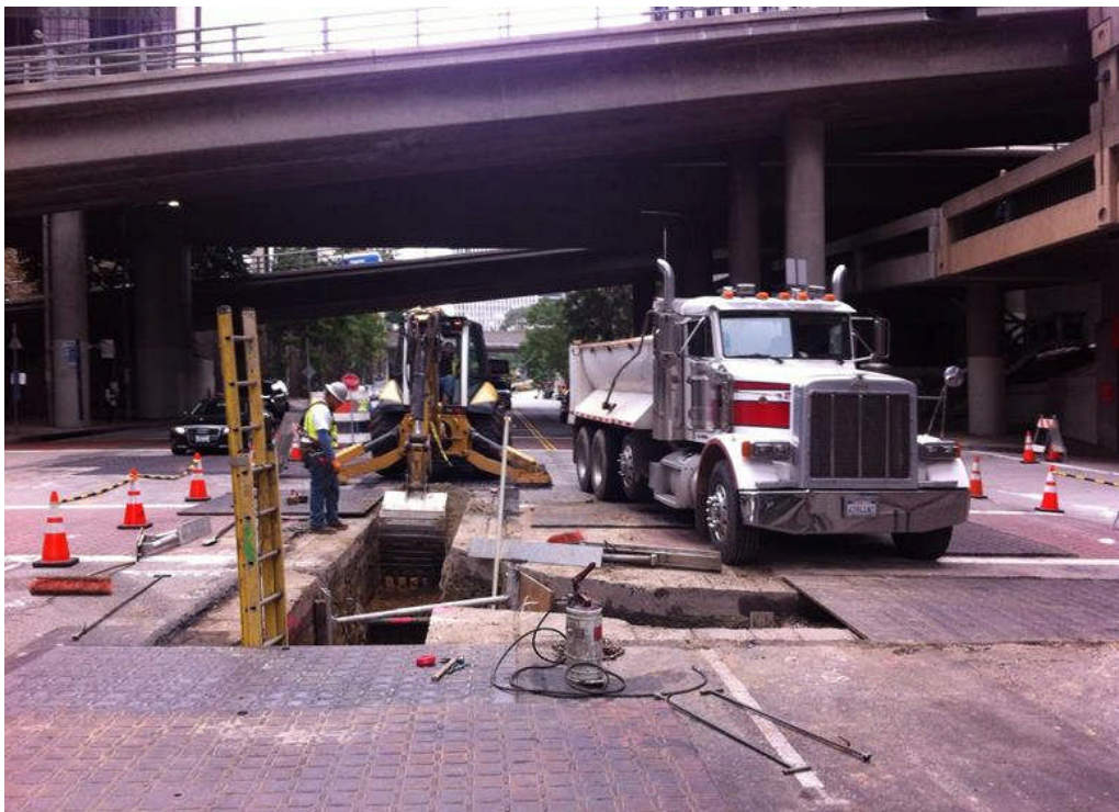
AUR C0981R – Shoring Installation at Flower Street
