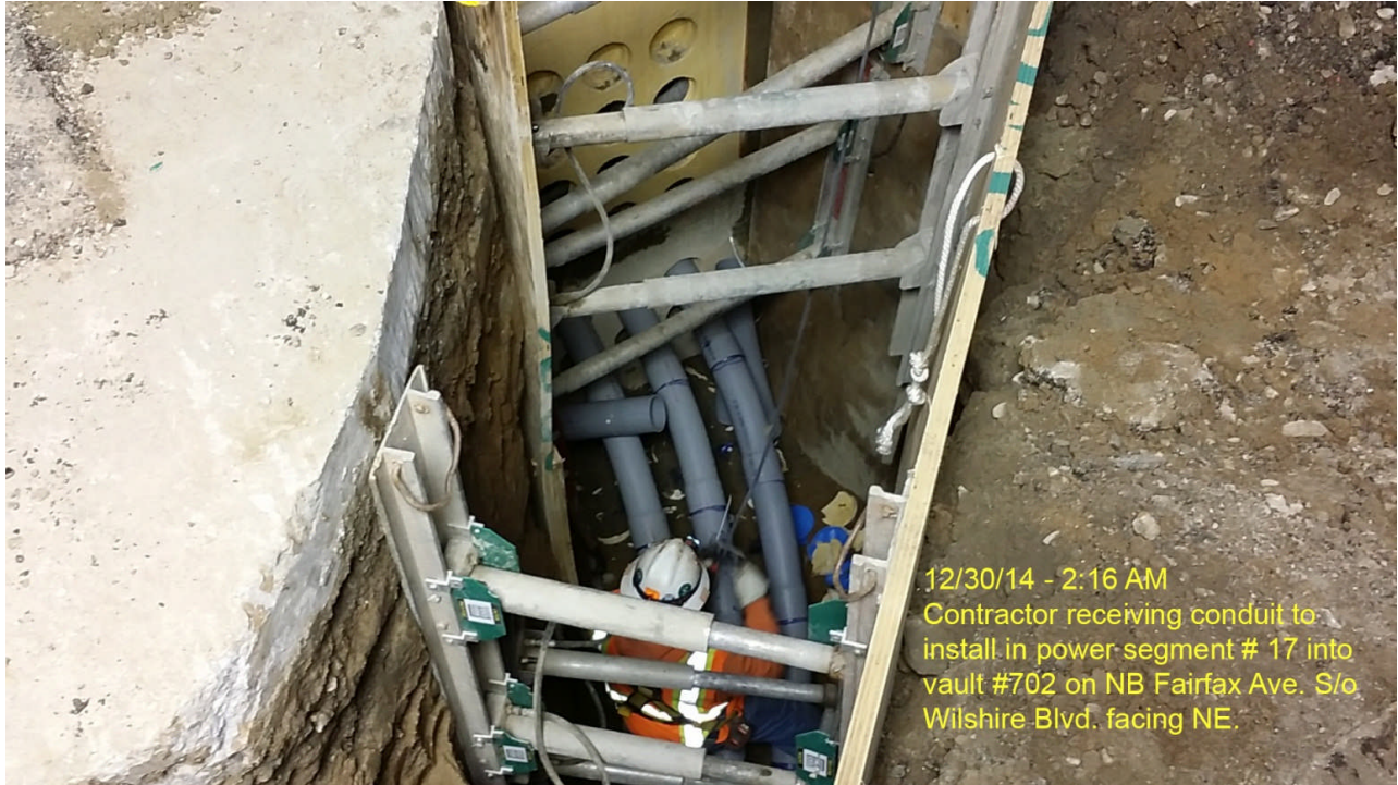
C1055 Contractor Performing Power Relocations
