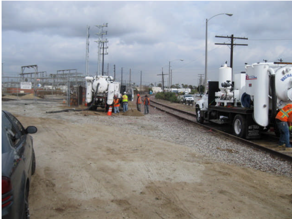
Potholing 138kv line north of Manchester.
