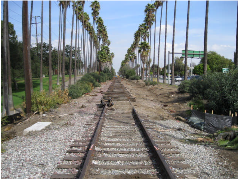
Rail removals north of Centinela.
