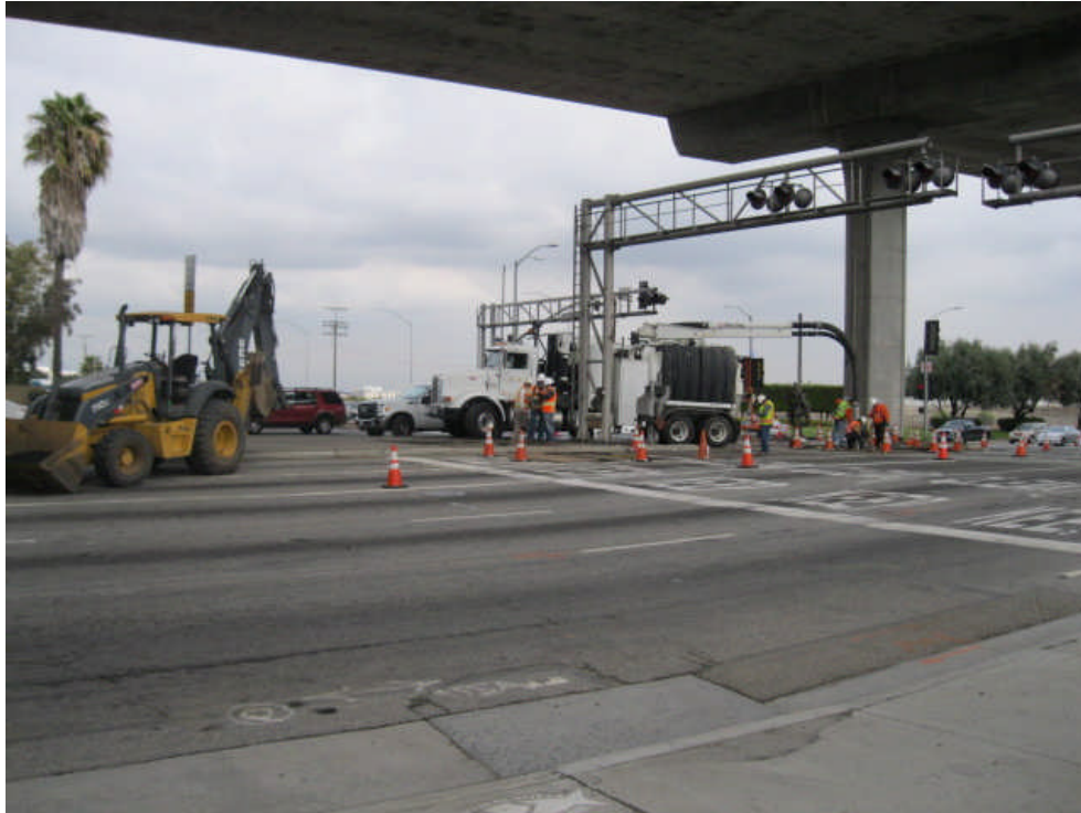
Potholing 138kv line at Imperial-Aviation Blvd.
