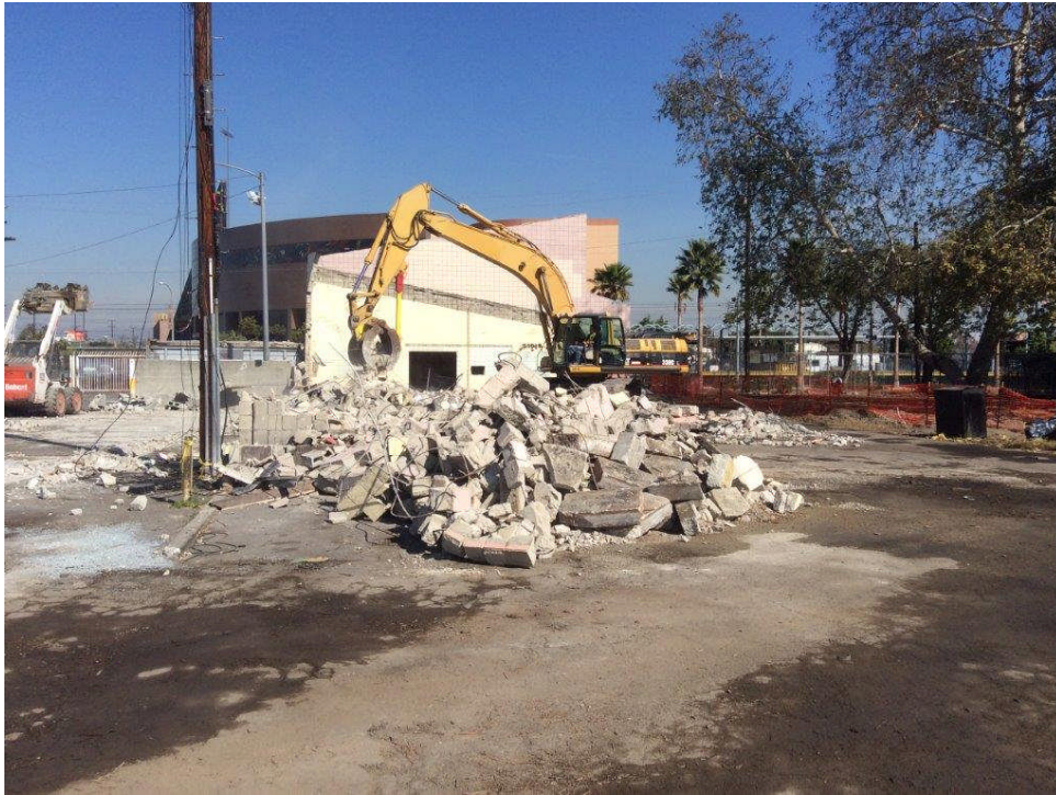
Demolition of existing structures at Crenshaw/Expo Station area.
