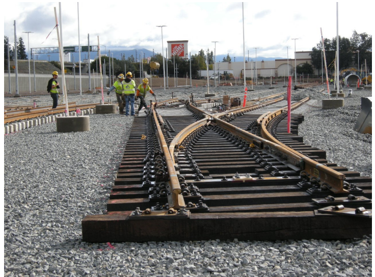
Segment 4: Continuing work on ladder track switches—lower NW Side
