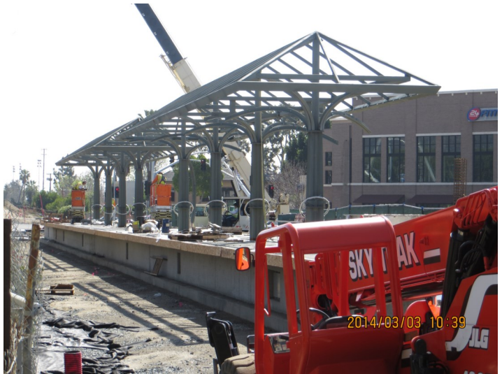
Segment 2: Arcadia Station Canopy Erection
