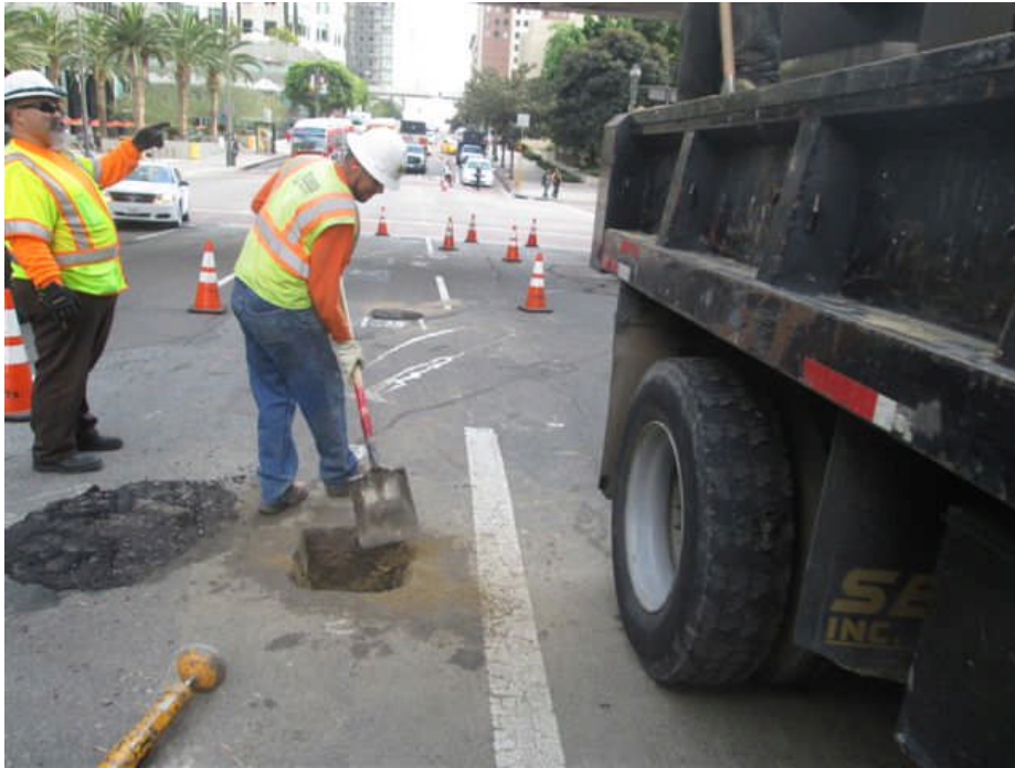
5 th Street and Flower – potholing of TWC facilities
