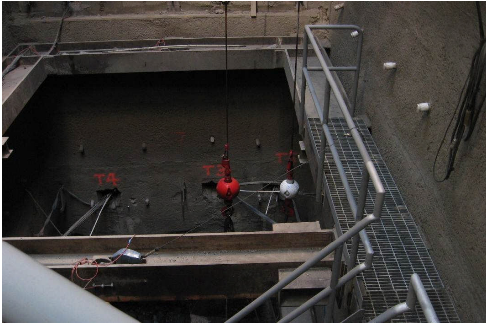
View of Exploratory Shaft 3 rd Lift of Waler Beams and Catwalk
