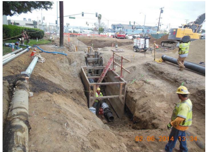
Segment 3: Waterline Work at Myrtle Avenue
