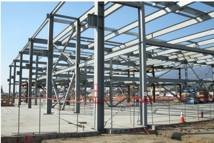
M&O: Main Shop Building Structural Steel
