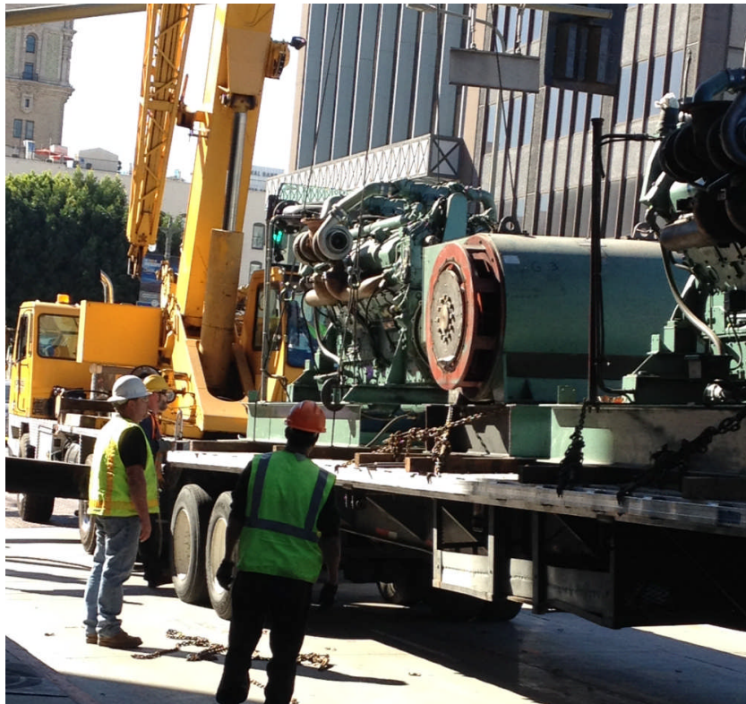
LA Times building generator removal
