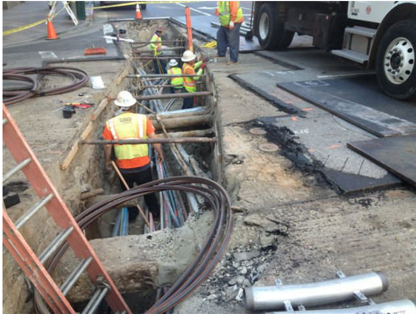
Flower Street and Sixth – Level 3 conduit installations by Irish Construction, Inc.
