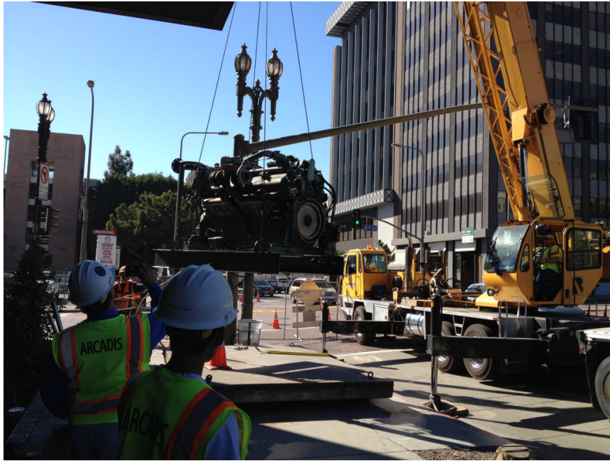
LA Times building generator removal
