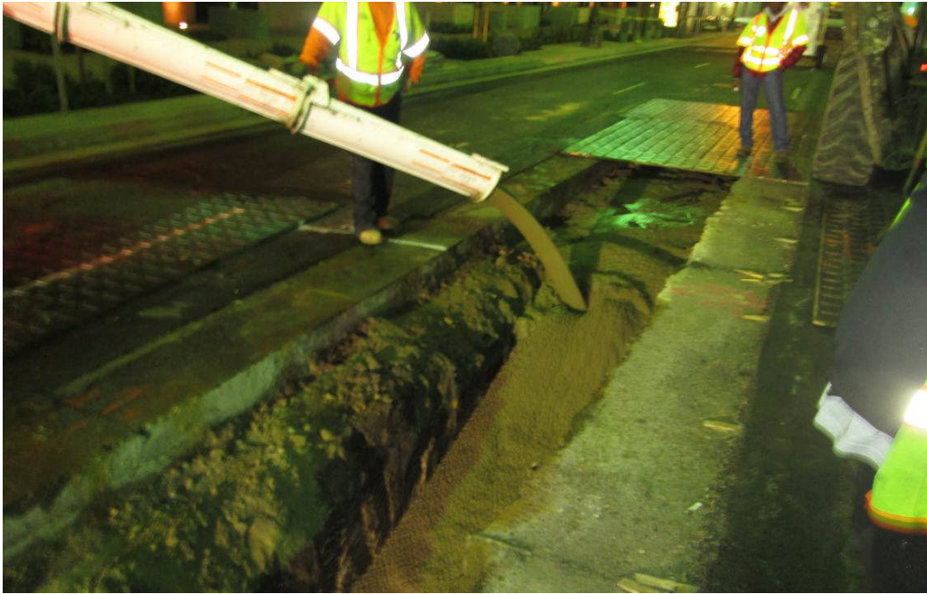
Slurry Backfill Over Utility Ductbank by the C1048 (Wilshire/La Brea) Contractor
