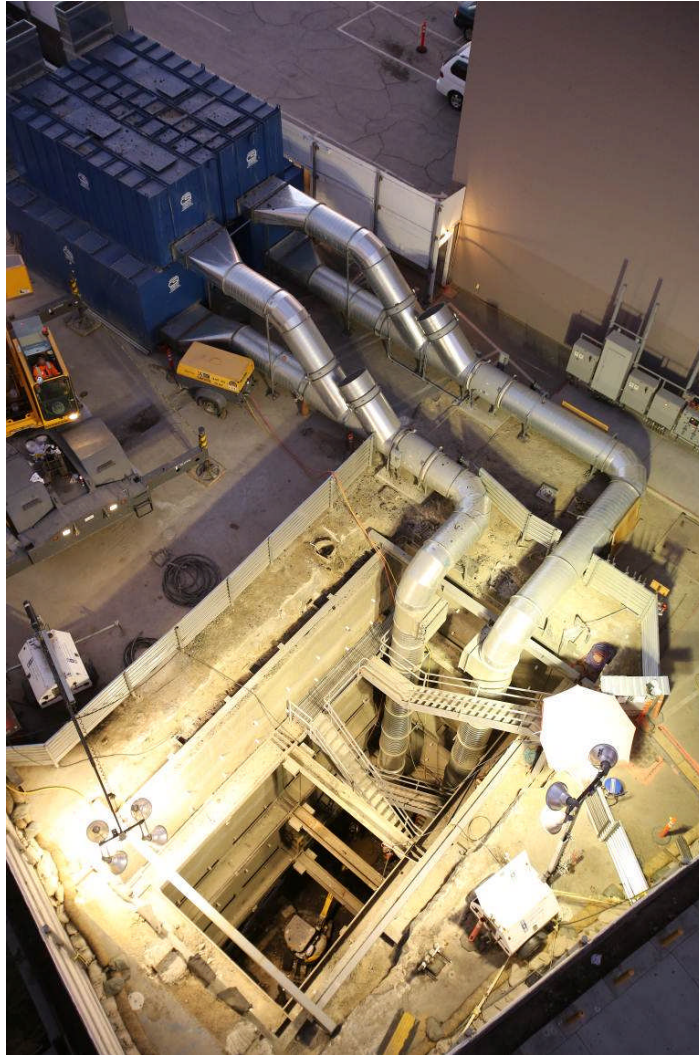
Exploratory Shaft Excavation Showing Three Levels of Steel Walers and Struts
