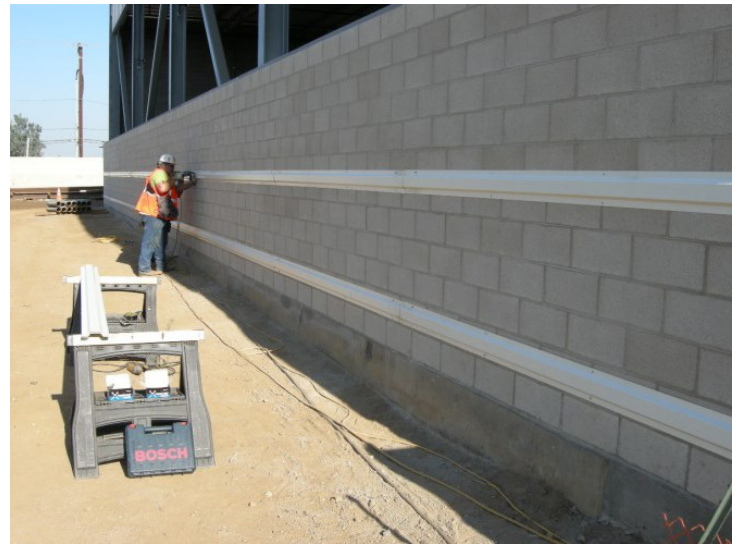
Operations Campus: Material Storage Building - Siding Installation
