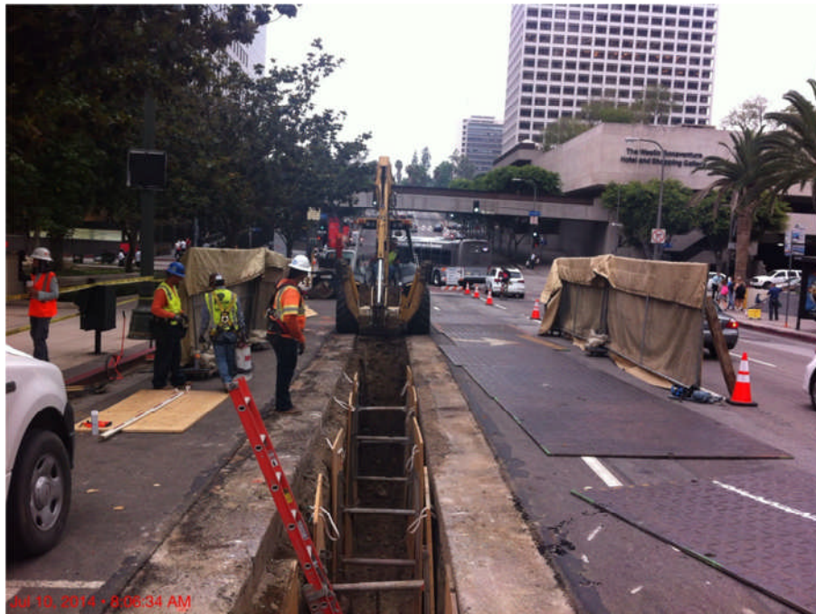
Trench excavation and shoring at 5 th St. east of Flower St.
