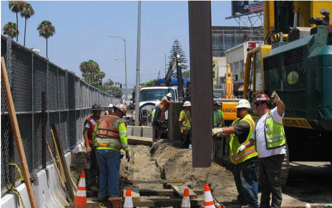
Lowering beam at pile located between MLK and Stocker.
