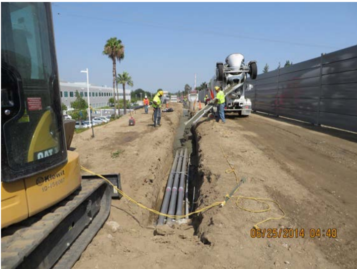
Segment 2: Ductbank work between Huntington and 5th
