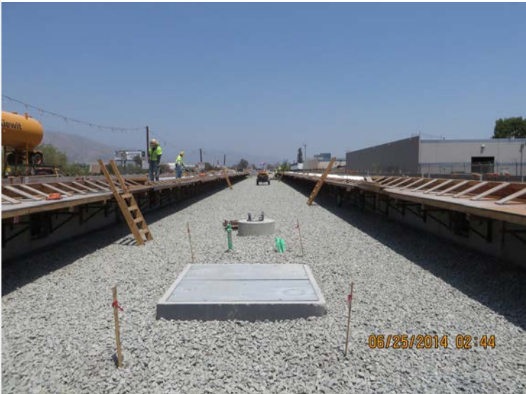
Segment 4: Irwindale Station - Deck Forming Work
