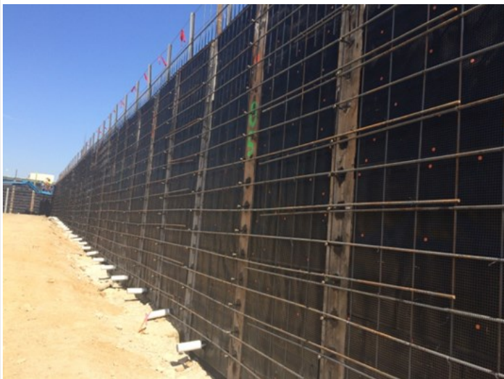
Rebar reinforcement for shotcrete walls at Azusa-Citrus Parking Structure
