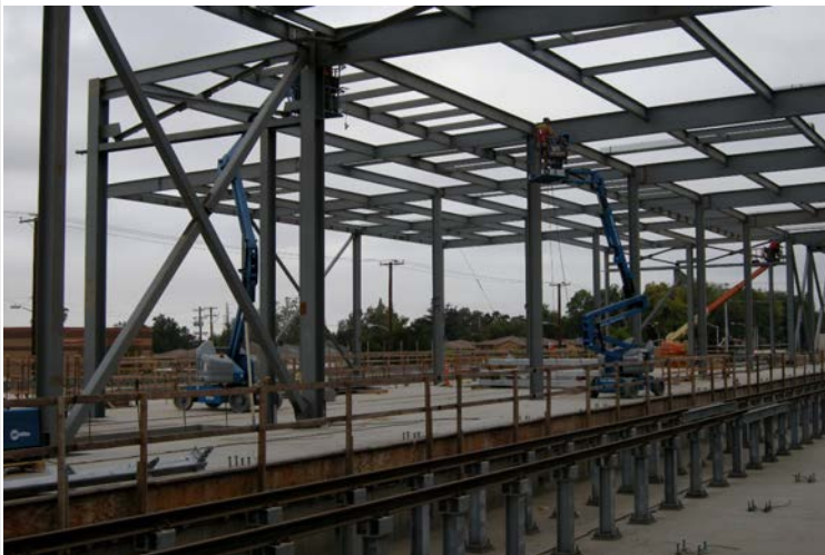
Operations Campus: Wheel Truing Shop - Structural Steel Work
